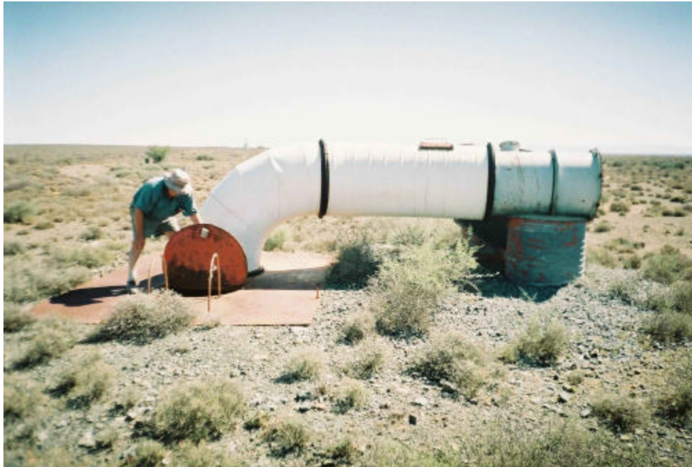
Figure 3.1.6 Disused ventilation pipe with unlocked trap door leading into Cameron shaft (no. 19 on location map).
