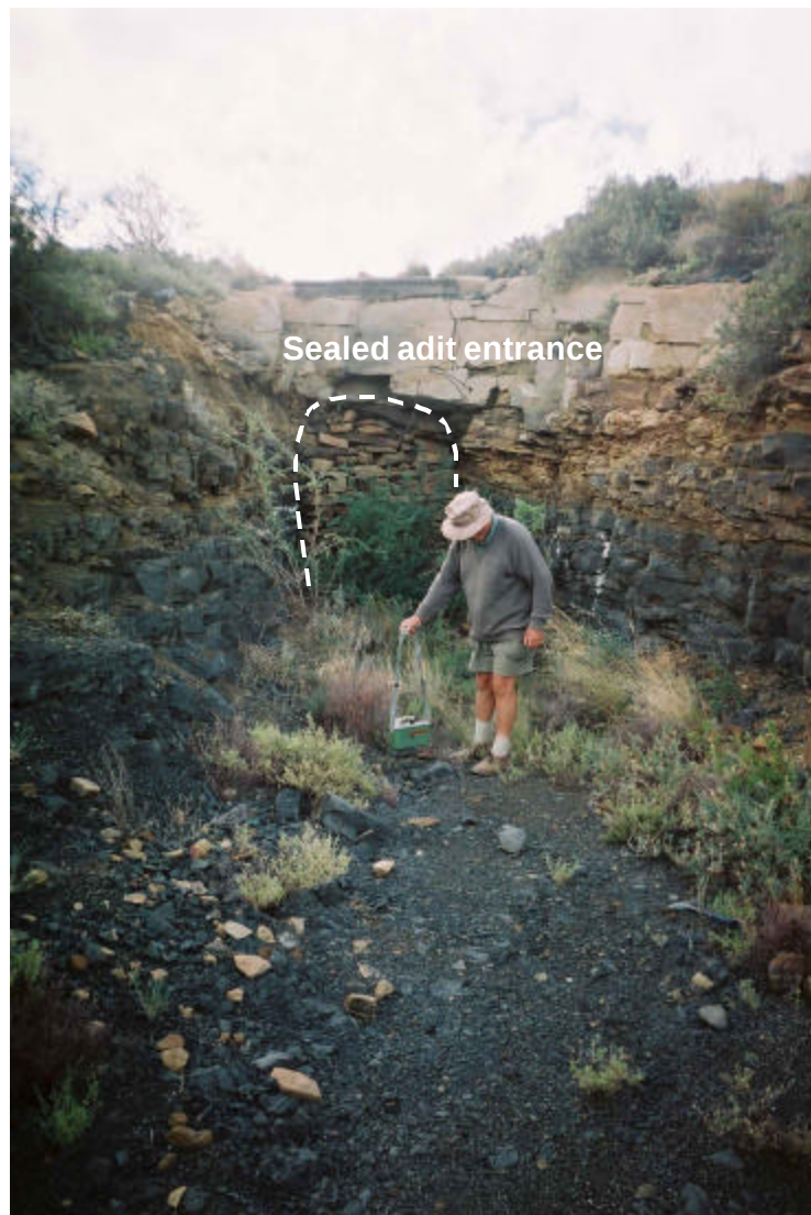
Figure 3.3.3 Entrance to sealed trial mining adit on DR-3.
