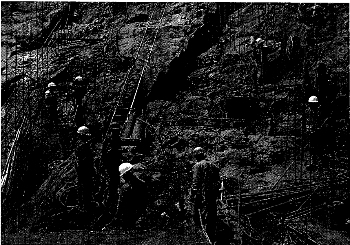
Figure 5.8-7: Compensation Foundation Reinforcement
