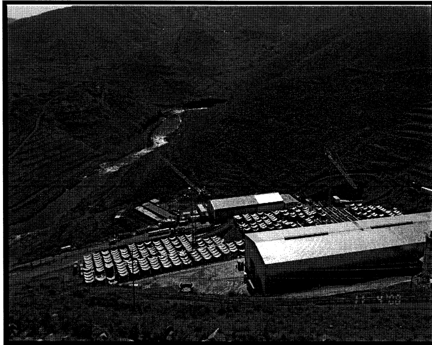
Figure 5.2-4: Medium flowing Senqunyane River. The Precast Factory of the Mohale Tunnel is clearly shown. Photograph was taken facing north from the contractors offices.
