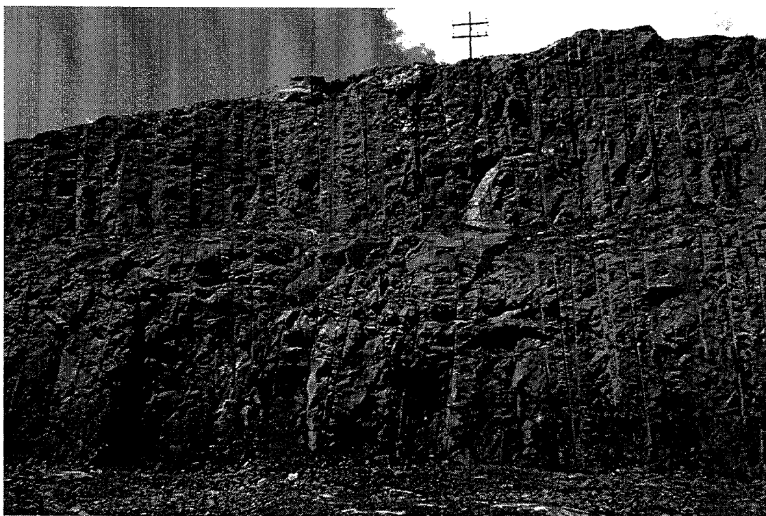
Figure 5.6-6: Right Abutment Access Road Cut. Two flows can be observed with some podsols lenses. This Photograph was taken facing southeast in Quarry 2.
