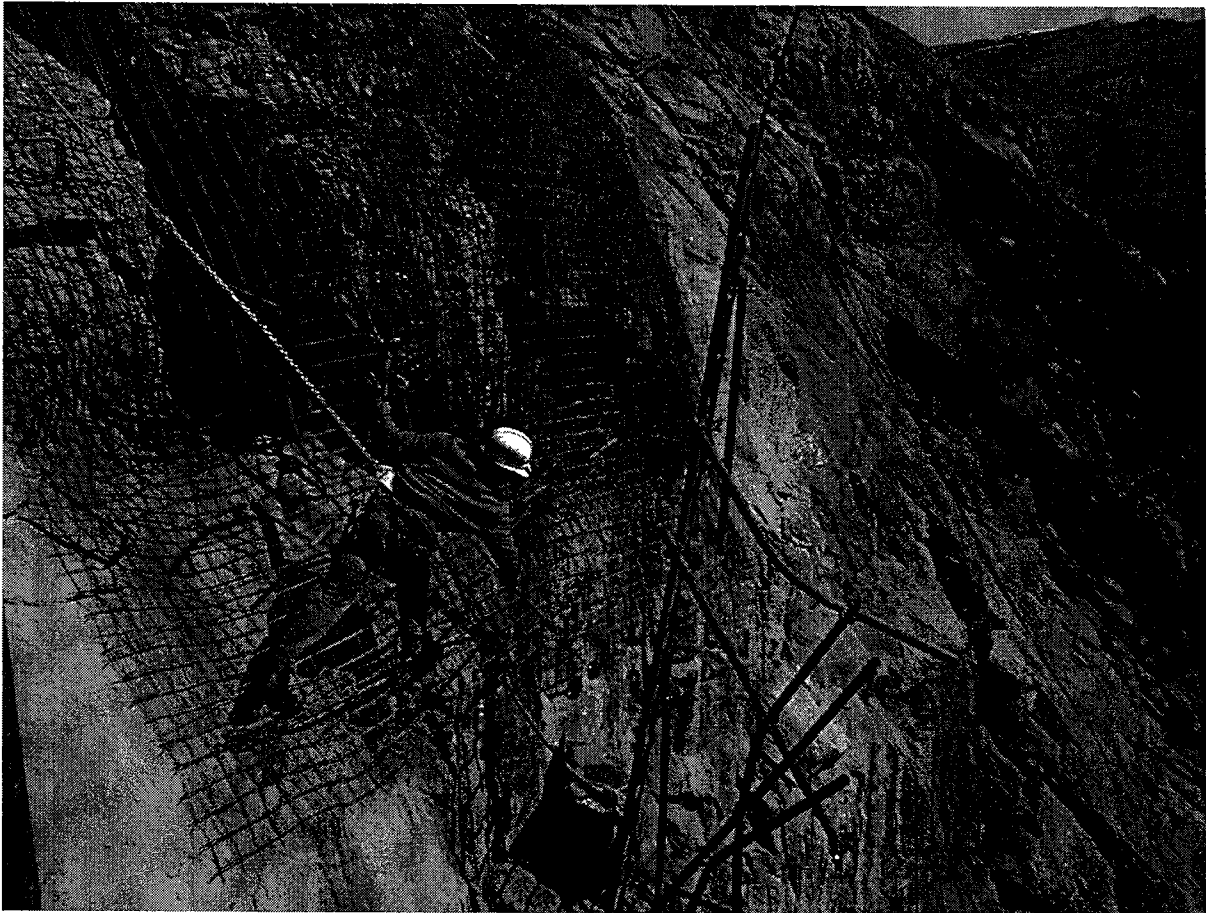
Figure 5.8-9: Laying Wire-Mesh. Work along the Slope next to Compensation
