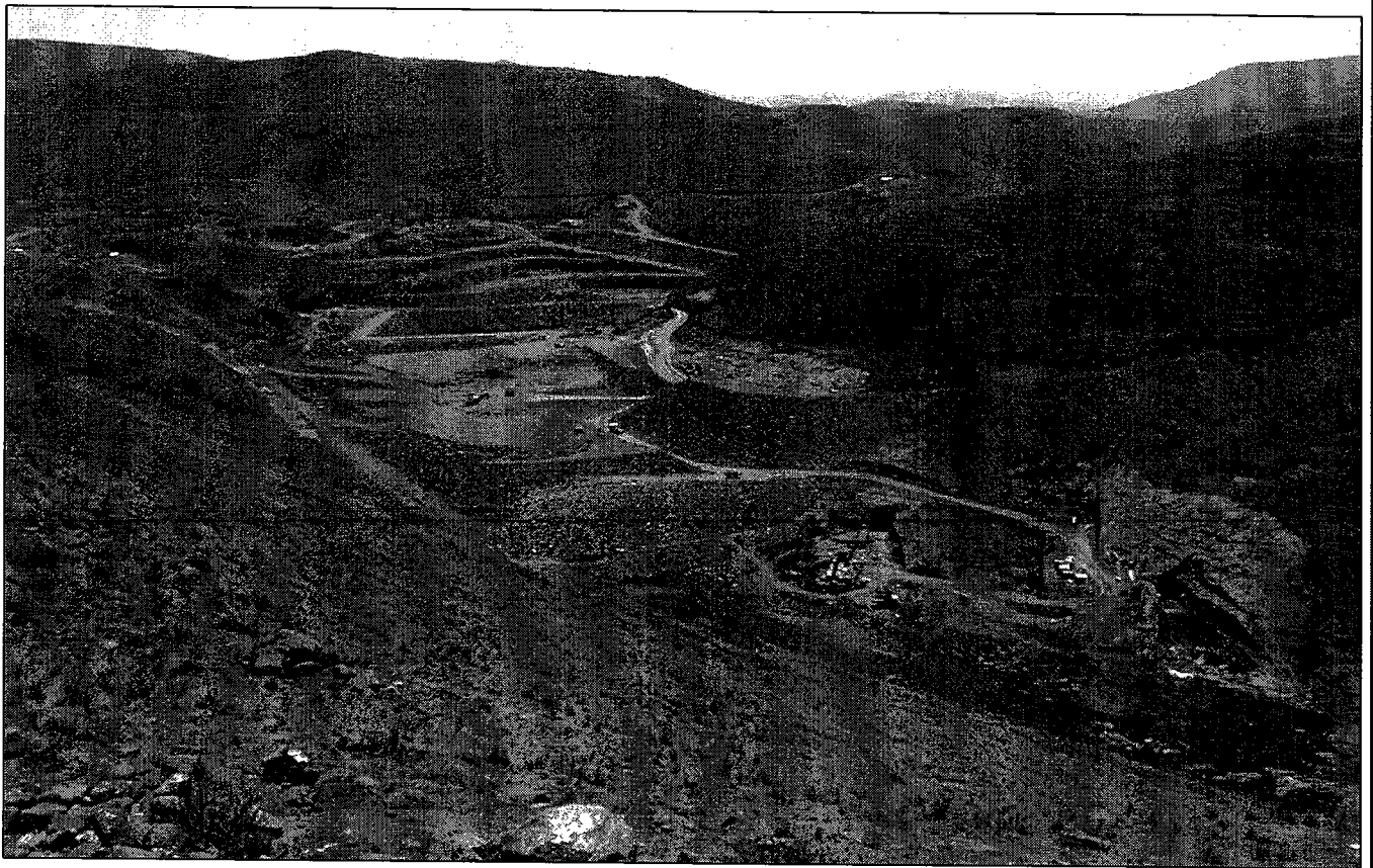
Figure 5.5-1: Dam Area and Quarry 1. Upstream Main Dam Site in Construction and Diversion Tunnel Outlets. Photograph was taken looking upstream from the Engineer's Office
