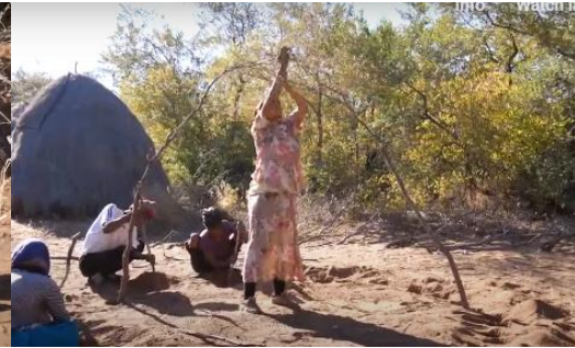
04 Loadbearing structures put in designated place
