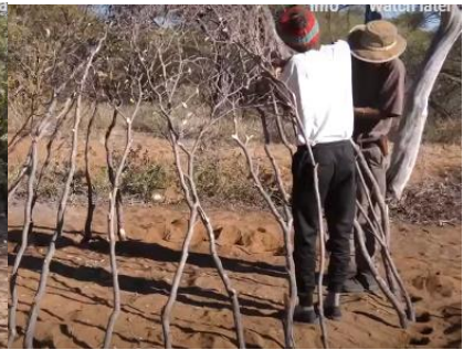
04 Loadbearing structures put in designated place
