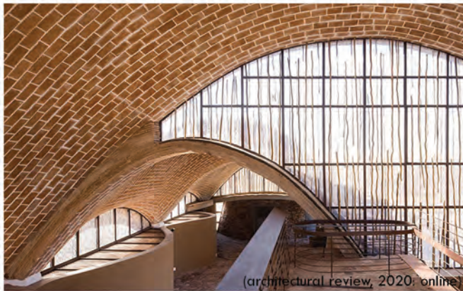
Figure 185: Spaces inside the interpretation centre
