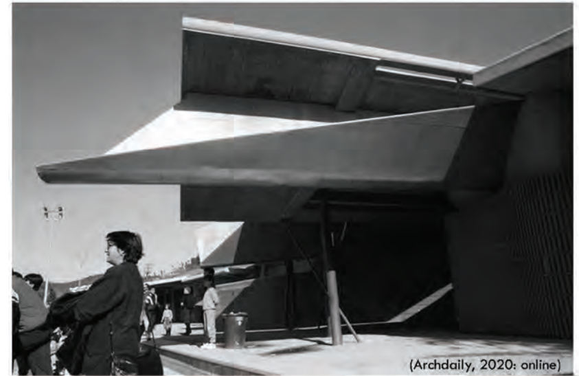
Figure 228: Archery pavilion gutter
