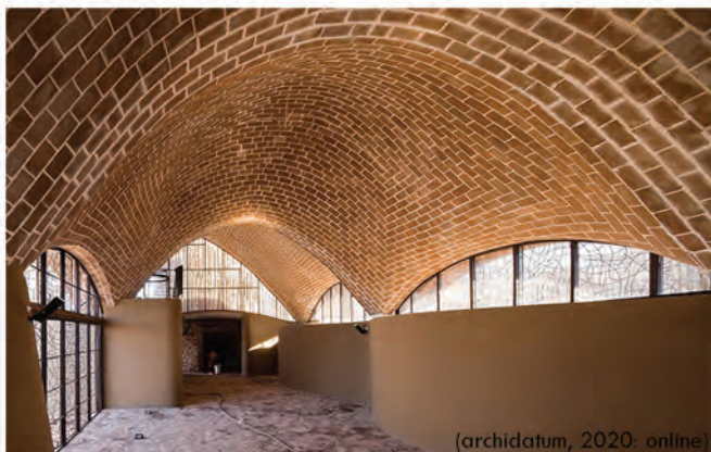
Figure 186: Spaces inside the interpretation centre
