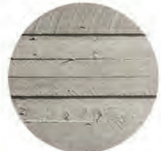
Boarded concrete walls
