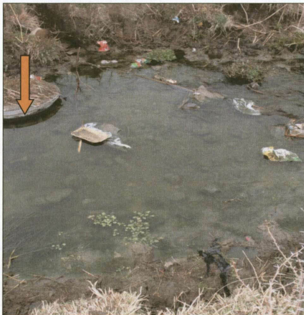
Figure 4.5: The upstream site in which a leaking manhole added sewage to stream water (Picture taken; January 2012)
