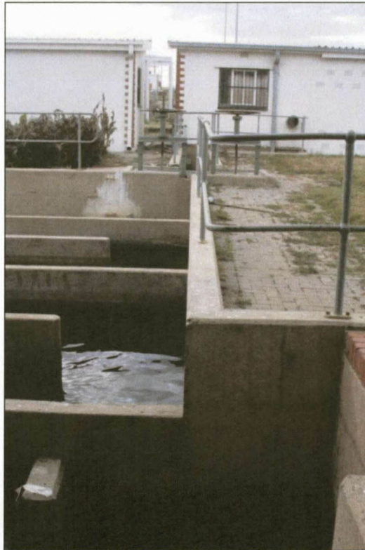
Figure 4.22: The white house is the chlorine house in which chlorine addition to the effluent happened (Picture taken; August 2011)
