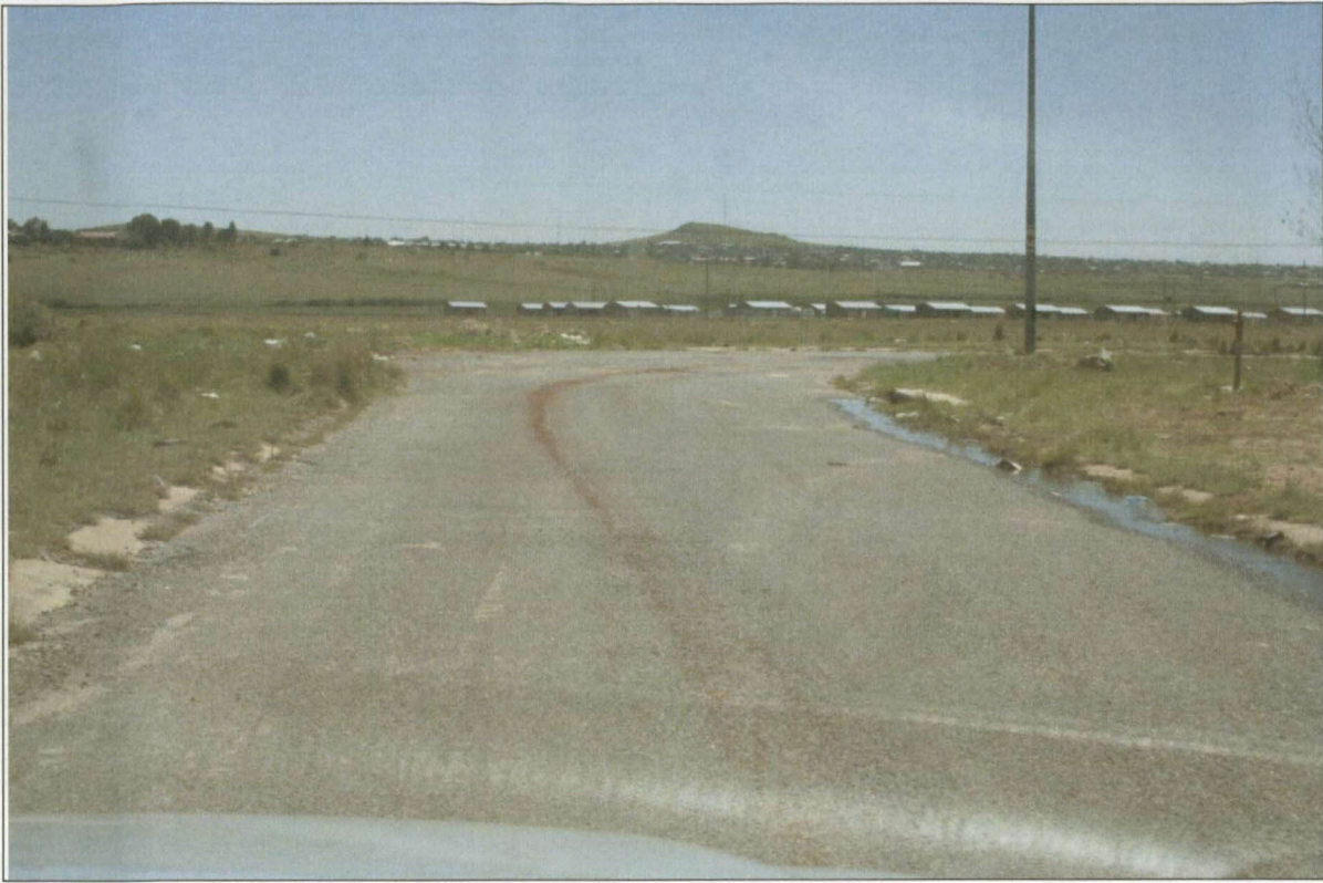
Figure 5.36: The line in the road is food dye that marked the continuous leakage of waste on the road (Picture taken: June 2012)
