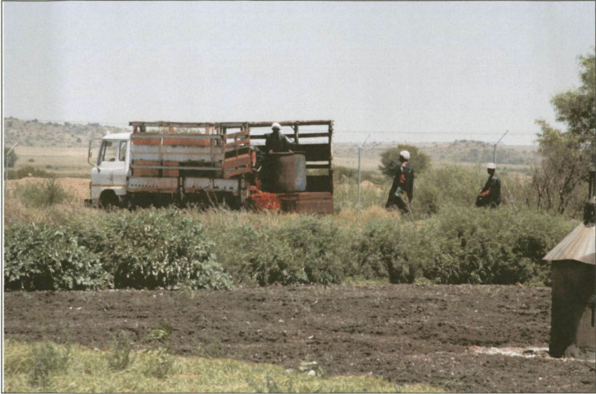
Figure 4.24: The sludge dam and an non-functional aerator (Picture taken: July 2012)
