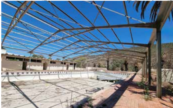
Figure 108: Current state of structure as viewed from entrance
