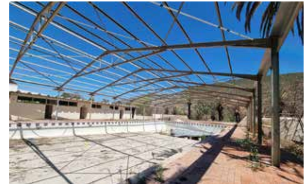
Figure 51: Existing structure. (Author, 2023)
