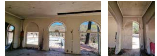
Figure 50: Interior of existing building. (Author, 2023)
