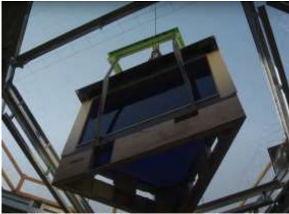
Figure 54 Australian Islamic Centre roof construction (wocomoCULTURE, 2019)
