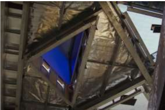
Figure 57 Australian Islamic Centre roof construction (wocomoCULTURE, 2019)
