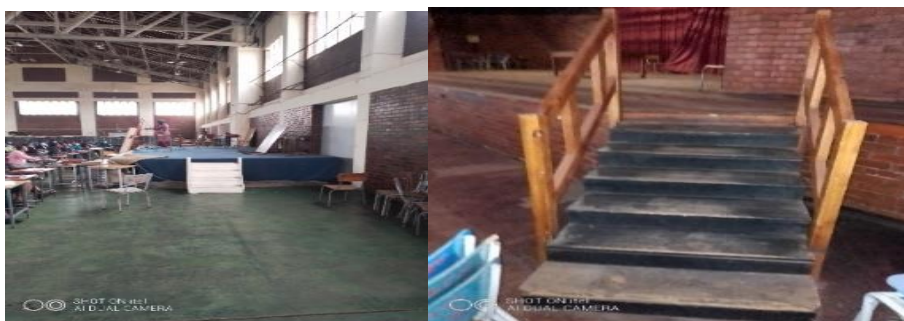
Figure 4.15: Steps used to access front stages in two of the lecture rooms
