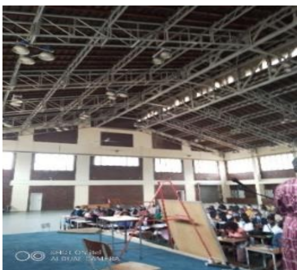
Figure 4.13: A lecture room with additional lighting
