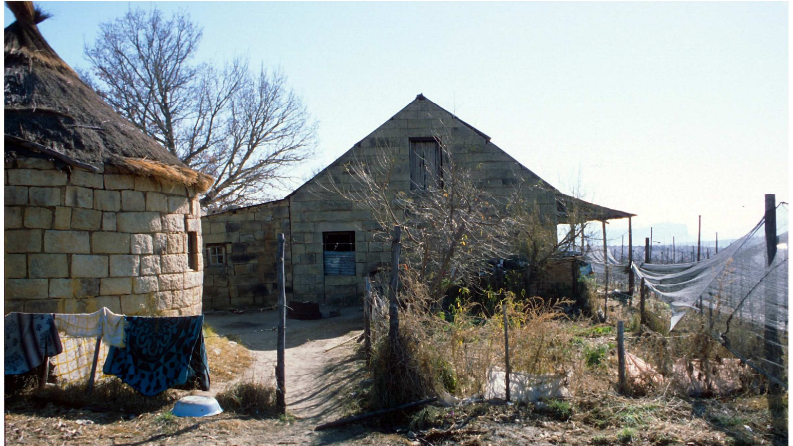
Fig. 63 Southern side of house and rondavel (1999)
