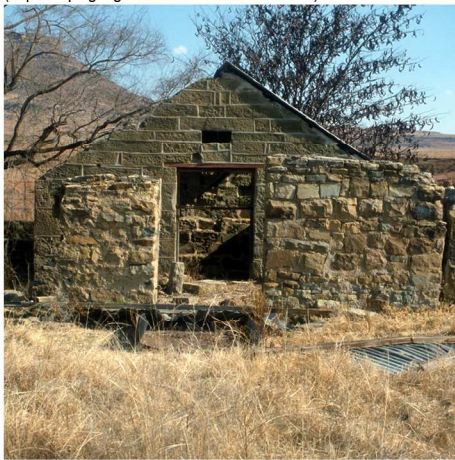
Fig. 128 Mill from the north-east (2000)
