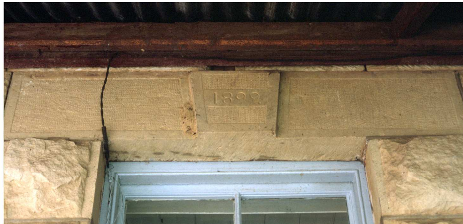
Fig. 244 Detail of original front door bearing the date "1899" on a raised and fielded keystone on the lintel. The house was only sill height when the Anglo-Boer War interrupted the building process. (1999)
