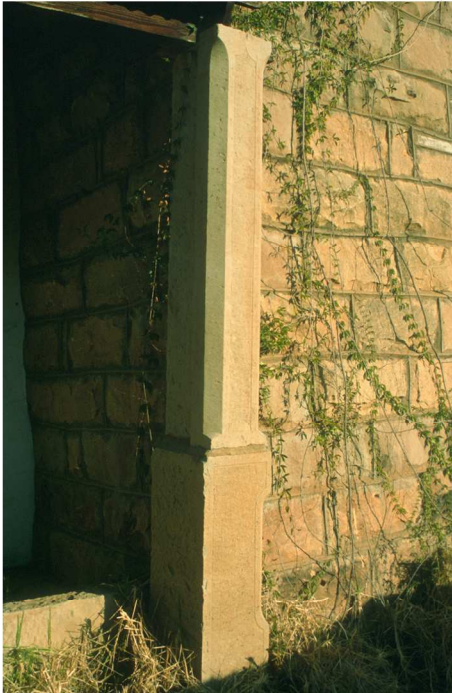
Fig. 74 Detail of a stoep column that survived from the first covered stoep. Details are more elaborate (chamfer and two different chamfer stops at top and bottom) than the newer columns. (1999)
