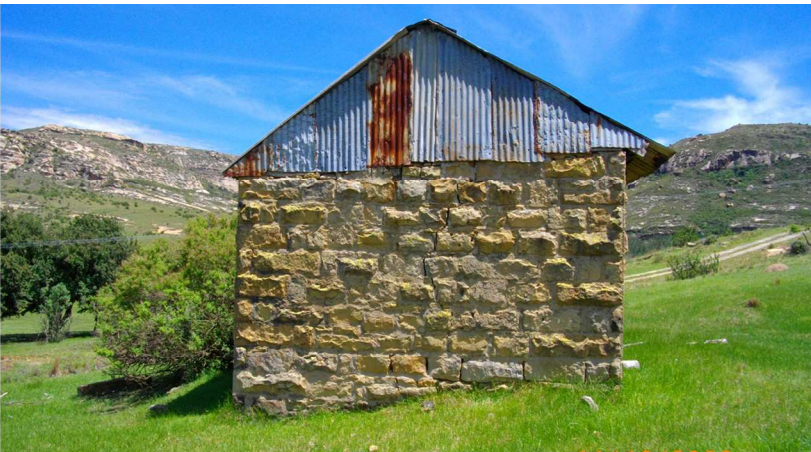
Fig. 192 South-eastern gable-wall (Photo: Louis du Preez 2012)
