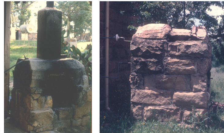
Fig. 309 & 310: Two hot water donkeys found during the survey. The farmhouse (left) at Bethel (1987) and (right) at Foutanie. (1987) Bethel and Foutanie were surveyed but not included into this collection.
