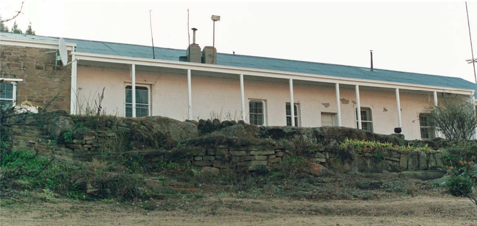
Fig. 140 South-eastern elevation, facing the Lesotho border. (2000)
