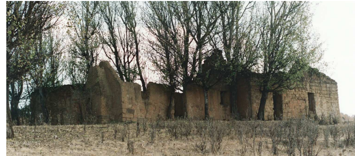
Fig.273 House Saunder (a farm manager's house) on Killarney, the Middleton Estate, where all additions were carried out with different building materials and techniques. The gable with the exterior chimney to the left is reinforced with sandstone on the corners, but mostly constructed with sun-dried brick. (2000)
