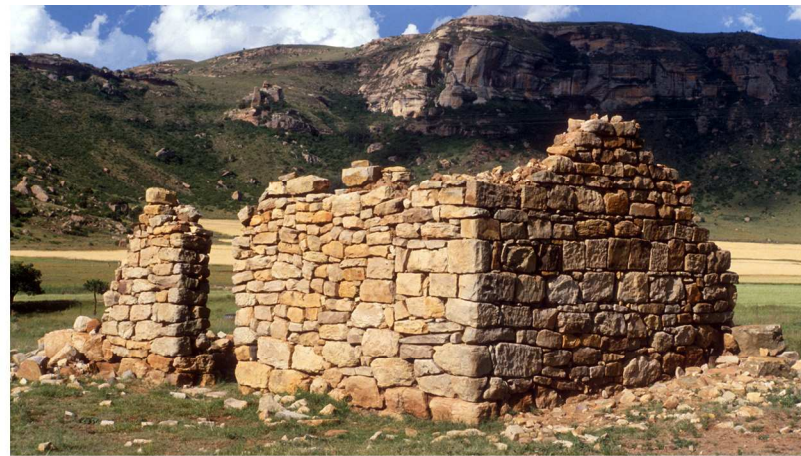
Fig. 10 The southern gable was built using a rough form of coursed rubble. The two long walls were of random rubble. The cottage might have been enlarged by just less than 1 m when the southern gable was rebuilt at some stage. (1987)
