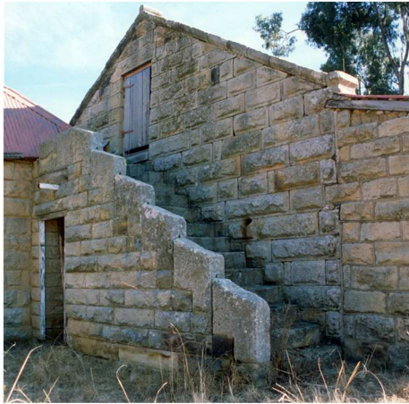
Fig. 198 Store under stone staircase leading to attic. (1999)
