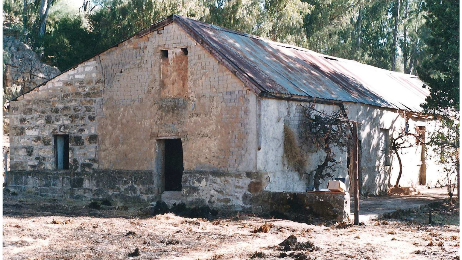
Fig. 156 Southern elevation showing the different additions on the gable. The door under the first gable leads to the stable. (1999)
