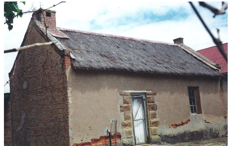
Fig 304 The kitchen as it was added to the back of Tierhoek, also with a huge hearth on the inside of the gable with the chimney as Schoonzicht. (Louis du Preez 1980)
