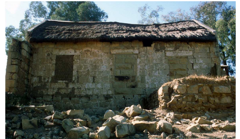
Fig. 181 Front of the phase 1 house which became more visible as the additions to the house disappeared. The door probably had a stoep in front of it, even if only to negotiate the steep terrain. (1999)
