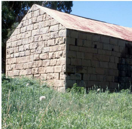
Fig. 251 Stable on the western side of farmstead, since demolished (1987)
