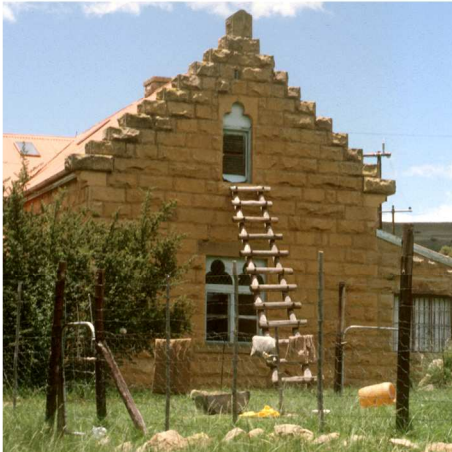
Fig. 38 Step-gable on north-western side of house (1987)
