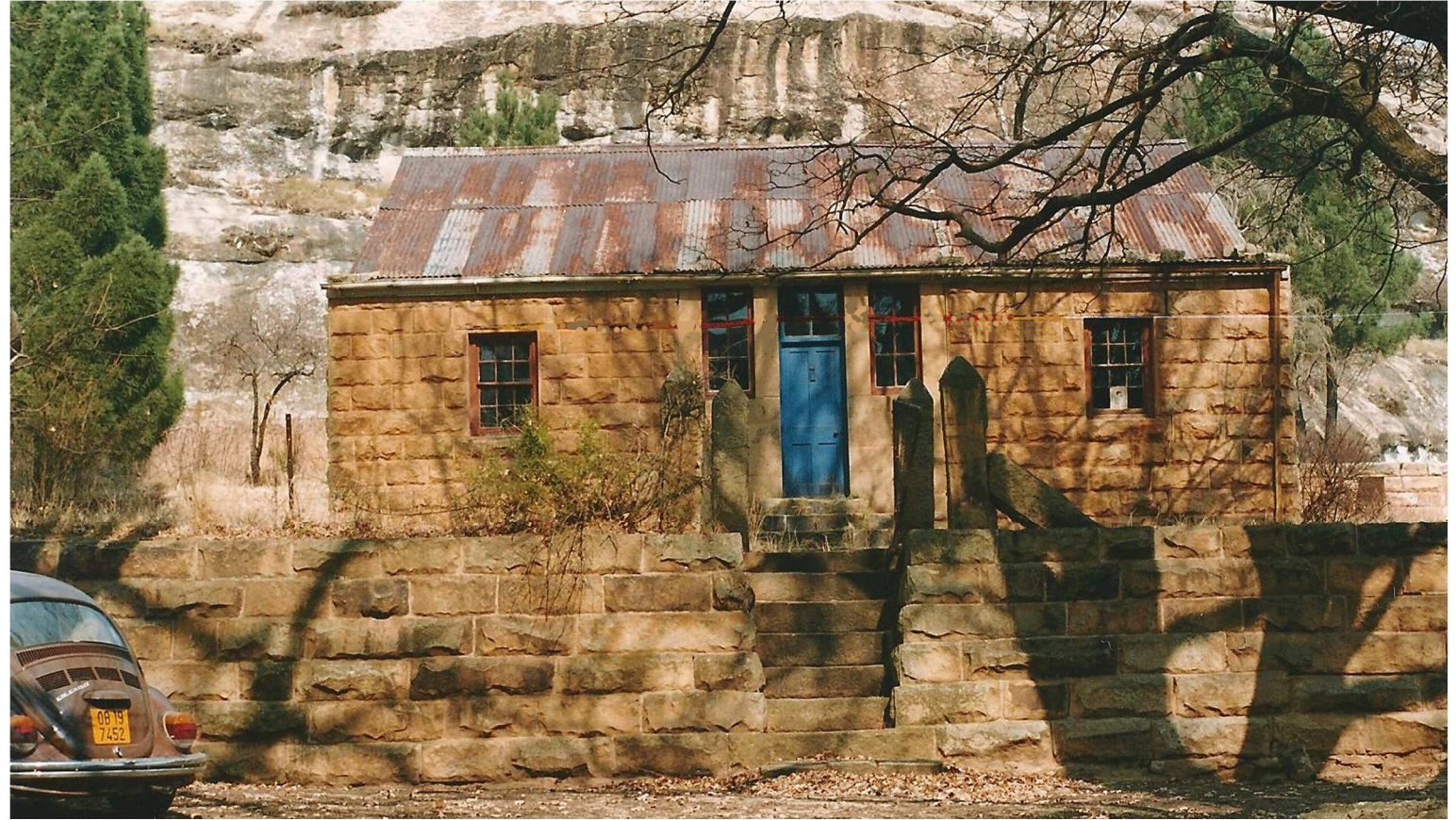
Fig. 24 Northern elevation showing the terraces that were constructed on the steep site. The front door and the two flanking windows might have the composition of a typical voorkamer entrance, but the original house had a passage to the living room. This door with windows were inserted when the covered stoep was enclosed. The room behind the sandstone screen is too small to function as a voorkamer . (1999)
