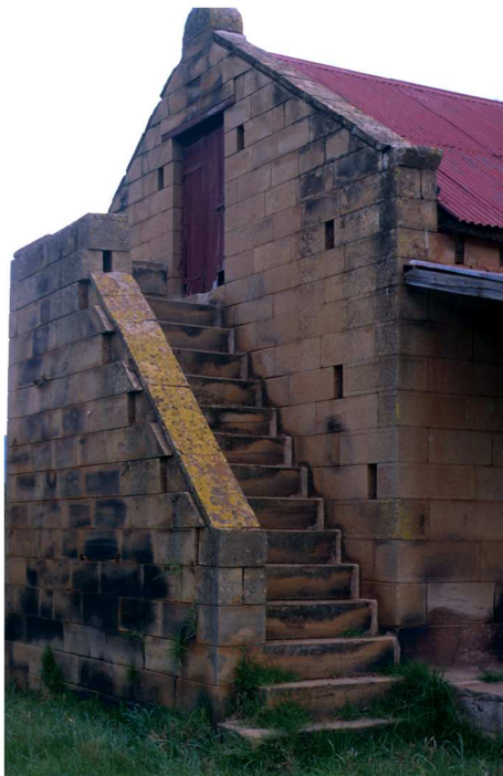
Fig. 211 Staircase on south-eastern gable. Note flush detailing of stonework. (1987)
