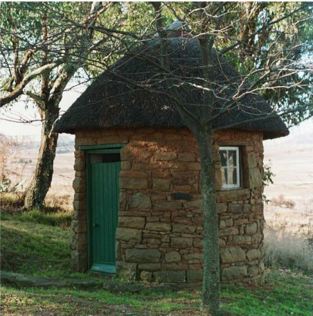
Fig. 139 Outside convenience (pit-latrine) for ladies with two seats inside. (2000)
