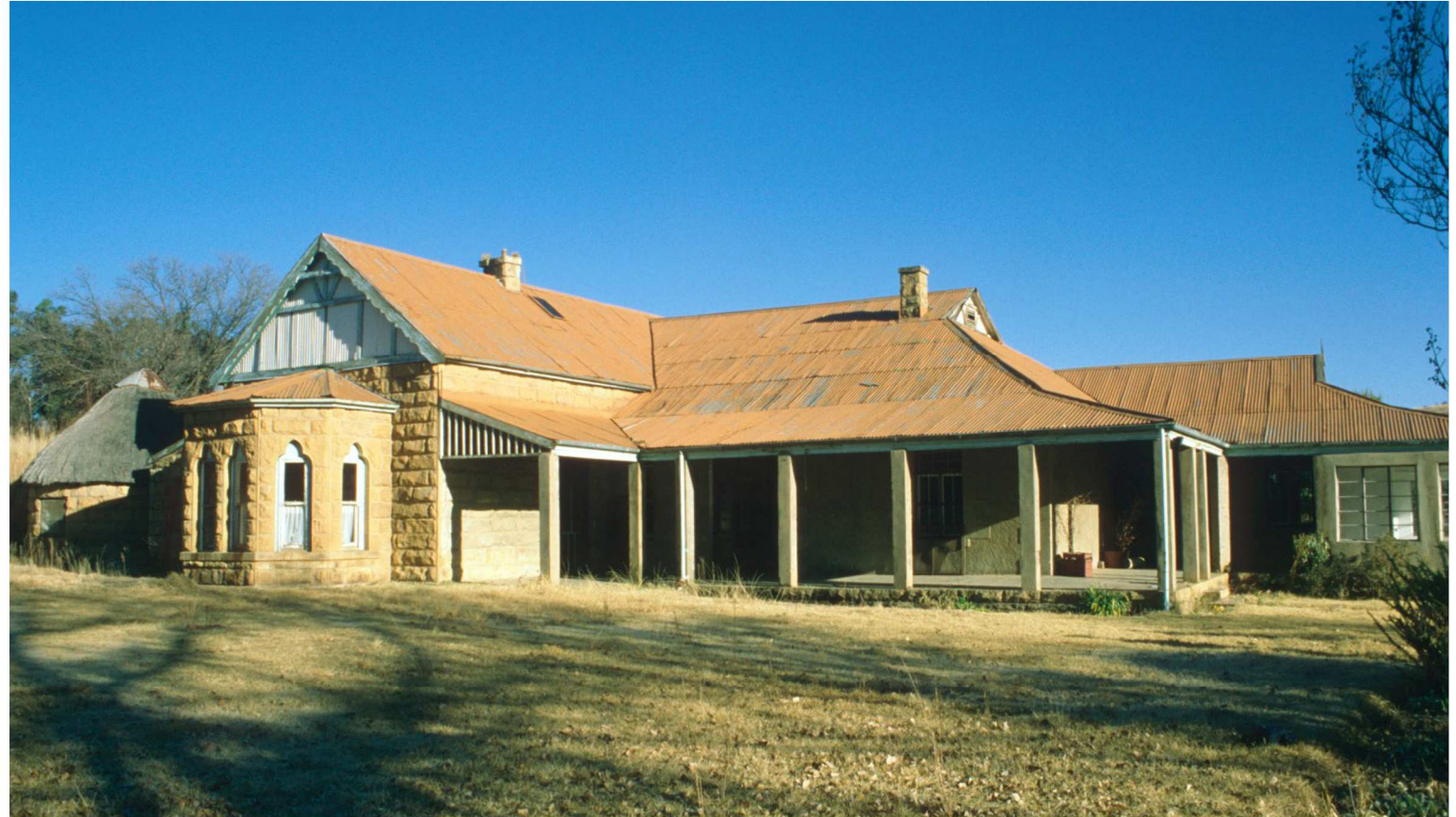
Fig. 41 South-eastern elevation of house and rondawel at left. (1999)
