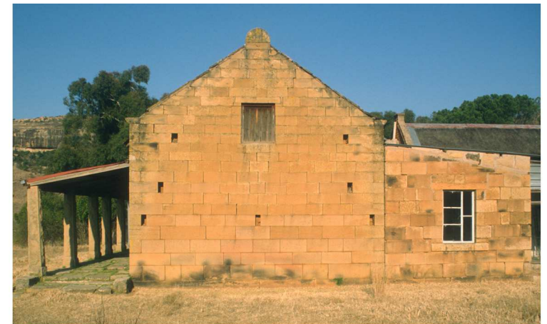
Fig. 215 North-western gable of the phase 1 house (1999).
