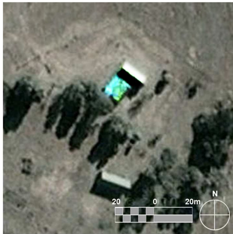
Fig. 220 Aerial photograph (scale 1:2 000) of House Fourie ( http://maps.google.com accessed 2011 08 18)
