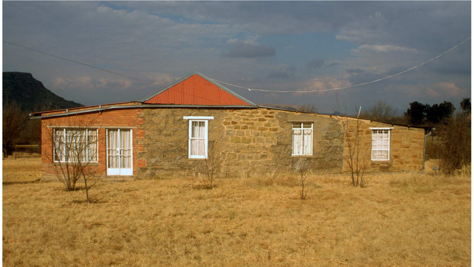
Fig. 106 North-western elevation towards the road passing on that side. (2000)
