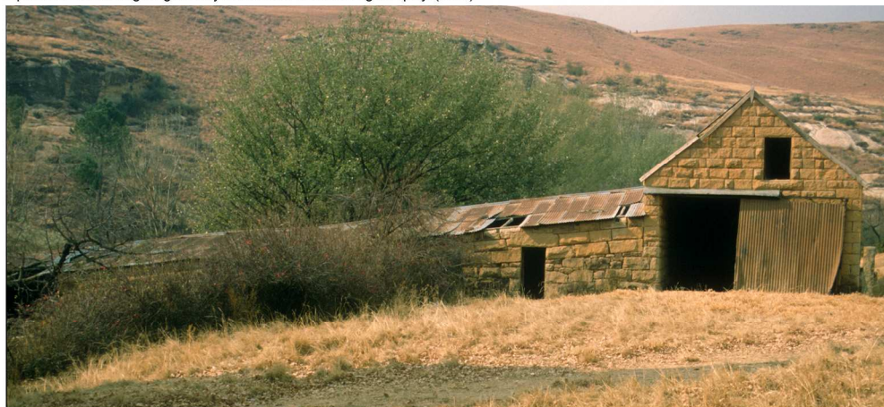
Fig. 36 The rest of the farmstead visible towards the east from the house. Note the dry set rubble kraal wall towards the left of the shed, with coursed ashlar on top of it, still following the gradient of the site. The door opening is set plumb in the wall - over-correcting slightly. (1999)
