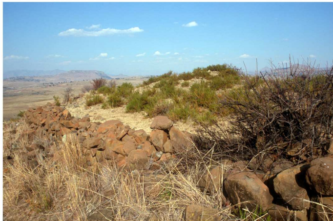
Fig. 117 The defences of Fort Campbell overlooking Lesotho in the background. (2000)
