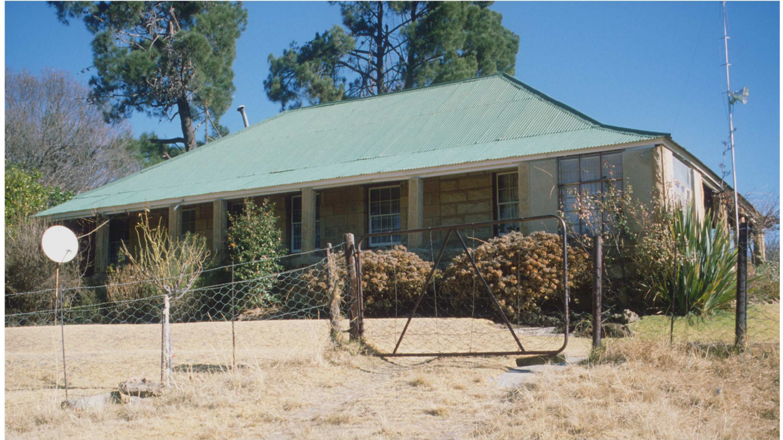
Fig. 96 South-eastern facade of the house showing the hipped roof with flared veranda on three sides. (1999)
