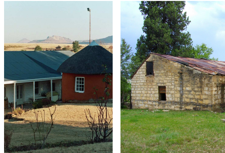
Fig.299 & 300 As soon as corrugated iron roof sheeting replaced thatch as roofing material, builders could adjust the pitch of the roof to a lower angle to accommodate the longer span of a double row of rooms. On the left is the Big House at Killarney (2000) and on the right is Modderfontein (1999). Both are examples of an extremely pragmatic approach.
