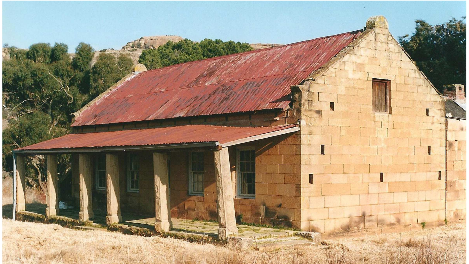
Fig. 213 Northern corner of House Fourie on Tierhoek. The flush finish of the walls contrasts with the rockface-with-smooth-arris-finish of the stoep columns (a monolithic stele on a base) that was added later to the structure. (1999)
