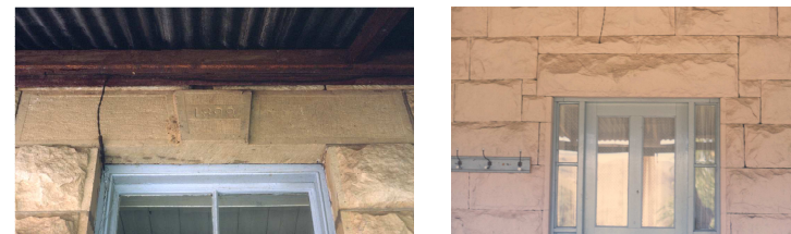
Fig. 279 & 280 Details of jointing and the alignment of lintels on Welkom. The house (right) and the old shed (left). (1987) & (1999)
