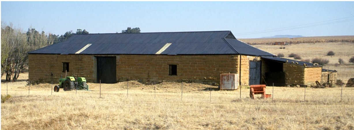
Fig. 149 The Shed seen from the east (2000)
