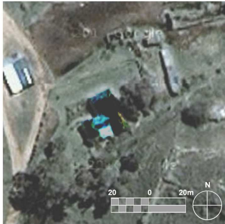
Fig. 81 Aerial photograph (scale 1:2 000) of Lusthof House ( http://maps.google.com accessed 2011 08 10)
