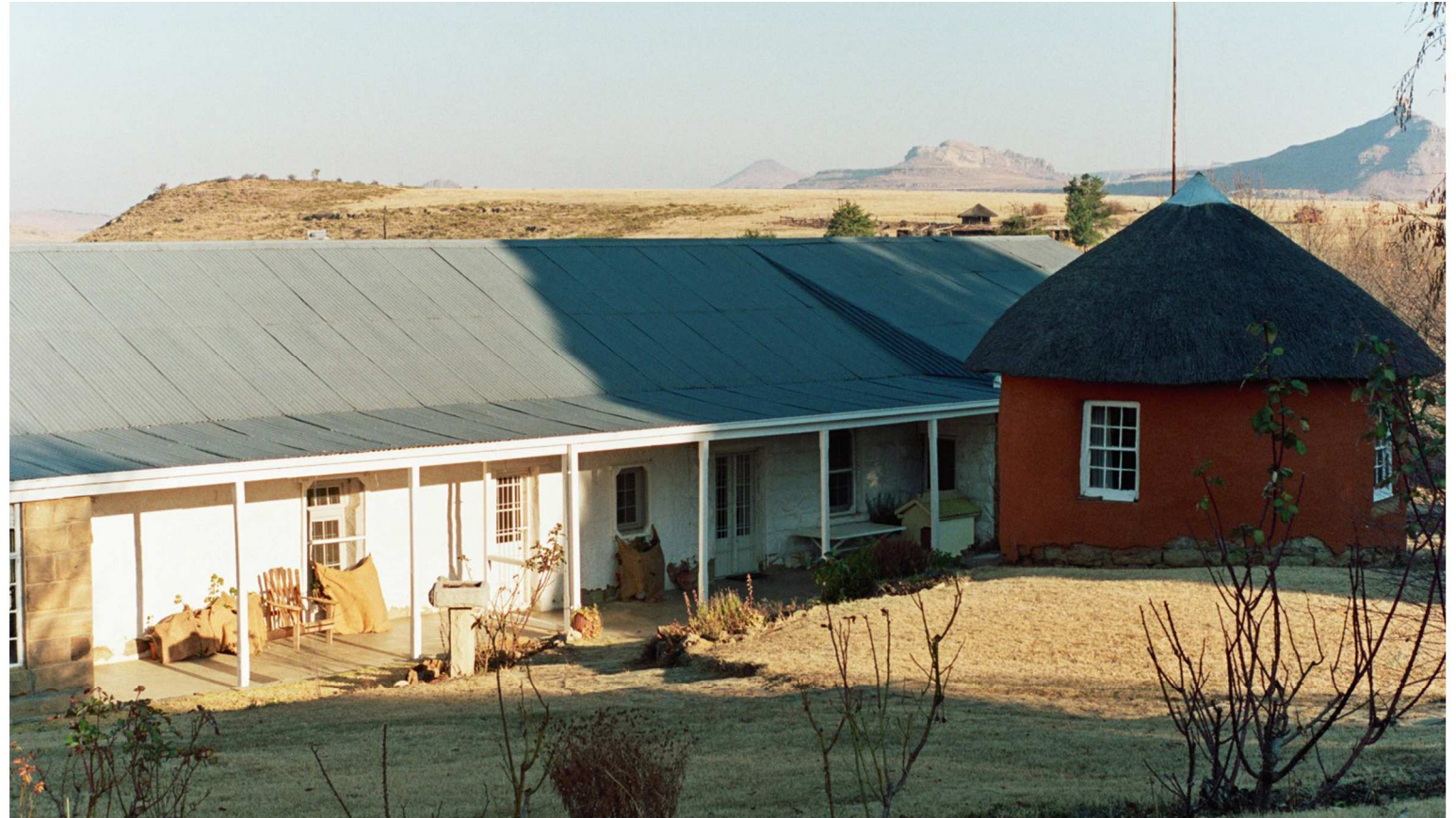
Fig. 141 North-western elevation showing stoep and double-doors to living/dining room. Note the pragmatic way in which different roofs of the different additions butt up against each other. (2000)
