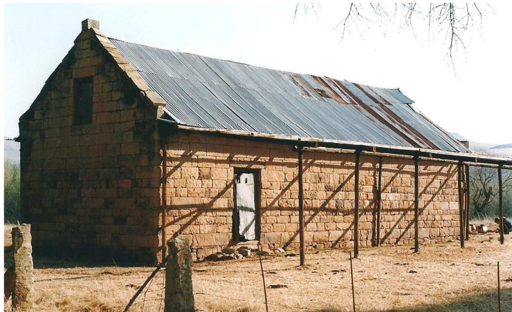
Fig. 226 The shed from the east (1999)
