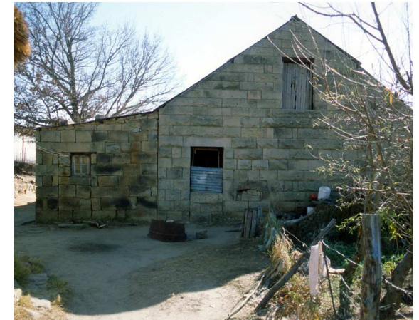
Fig. 65 Southern facade of house showing the joint between phase 1 and 2. (1999)
