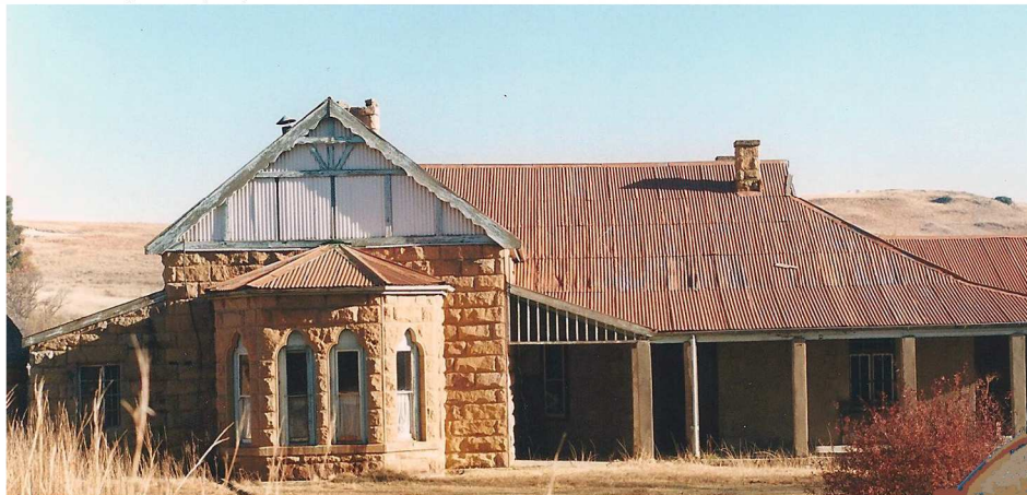
Fig. 59 The bay window towards the south-east with corrugated iron sheet infill in the gable above and fretted fascia. The house has a fully developed gabled hip roof with flared veranda to the north-eastern side (right). (1999)
