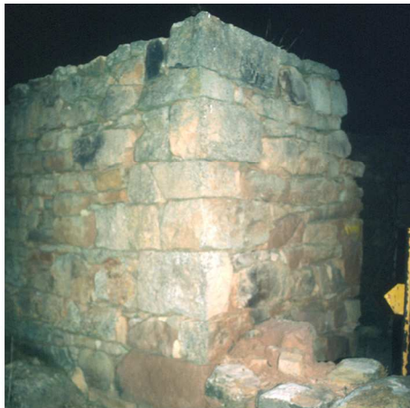
Fig. 87 Southern corner of Outbuilding (1999)
