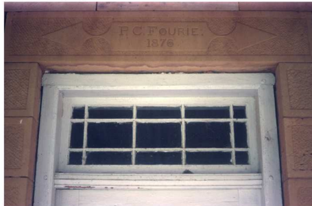
Fig. 221 Detail of fanlight and architrave over front door with the inscription "P.C. Fourie. 1876." (1987)
