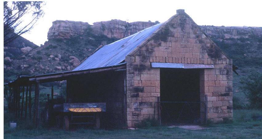
Fig. 227 The shed from the north (1987)
