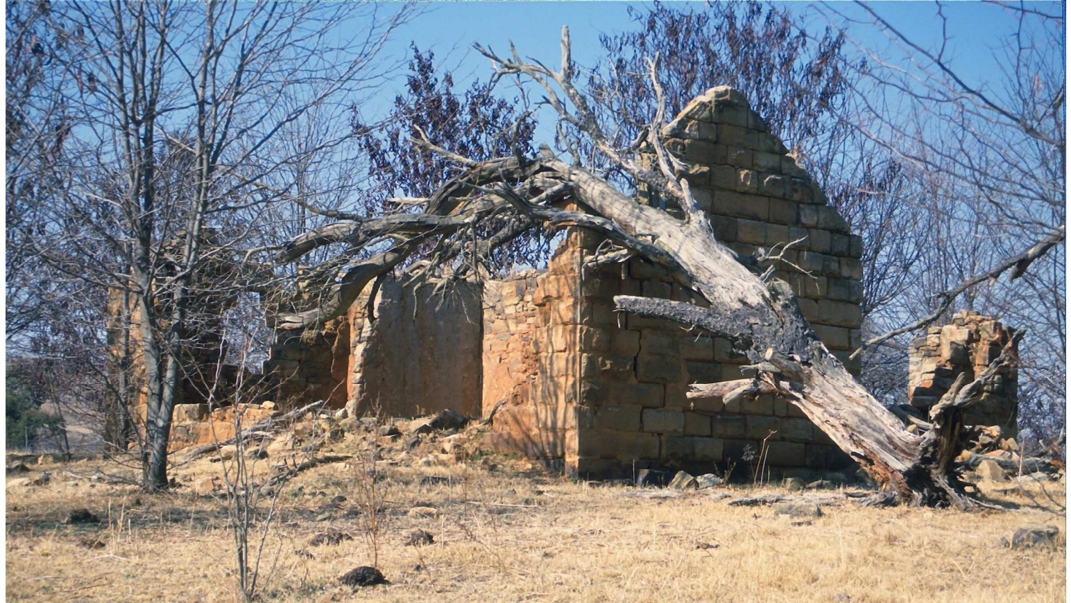
Fig. 118 The Miller's House as seen from the mill, the north-west. (2000)
