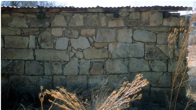
Fig. 229 Detail of back of Toevertrouw cottage showing more than 10 of the re-used gable stones. (1987)
