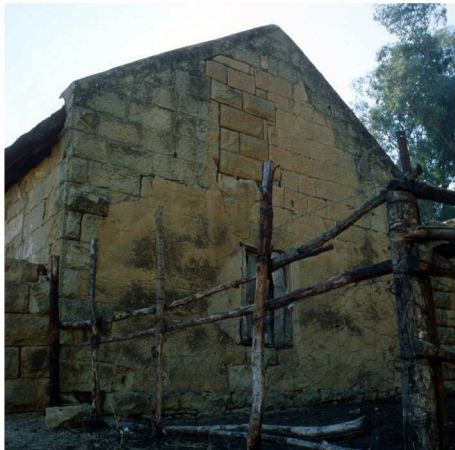
Fig. 178 Detail of south-western corner of house with quoin-stone detail and light plaster still visible of phase 1 house. (1999)
