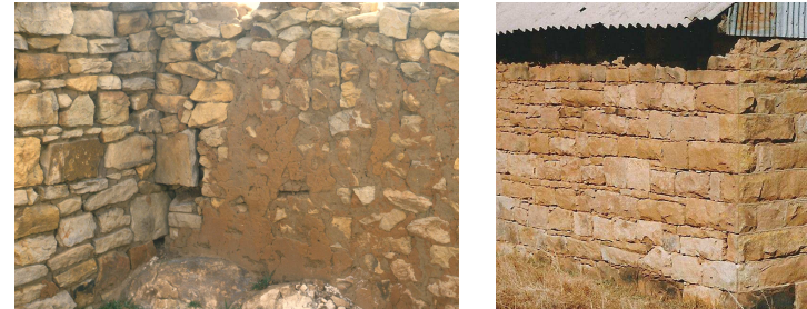
Fig. 275 & 276 On the left is Bethlehem Star Cottage showing random work and coursed random work. (1987) On the right is Present Poort Second House with coursed random work and ashlar on the corners. (1999)
