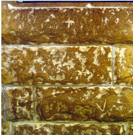
Fig. 57 Mason's marks ("V" or "+" etc.) on the sandstone blocks identifying the stone cutter (1987)
