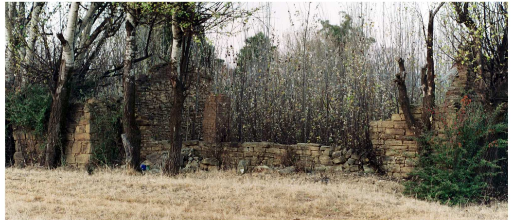
Fig. 108 Smithy as seen from the west. The chimney is at the centre of the photograph. (2000)
