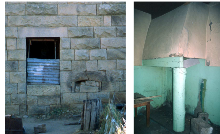
Fig. 301 & 302 The bakoond opening next to the back door at Kransfontein dating from 1885 (left) and (right) the hearth with the massively built hood inside the early kitchen at Schoonzicht dating from 1883. (1999)
