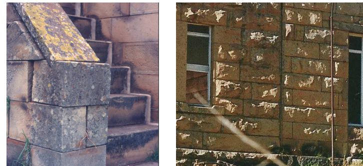
Fig. 277 & 278 Detail of the jointing at Tierhoek House Fourie on the left. (1987) The old shed (right) on Welkom is on the right. Note the shift in course depth between the shed and the addition. (1999)
