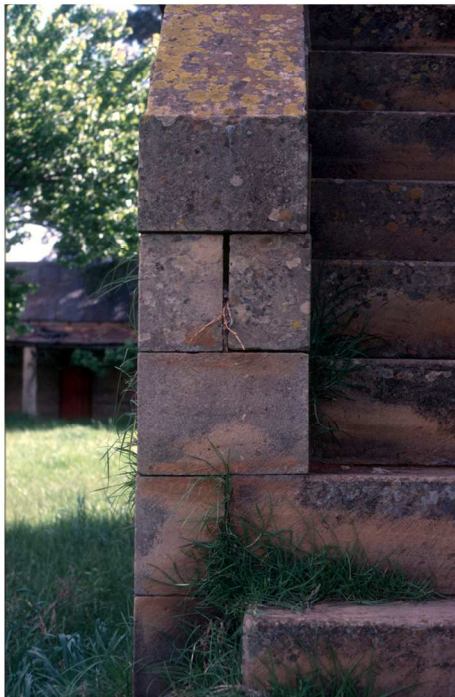
Fig. 212 Detail of balustrade in sandstone (1987)
