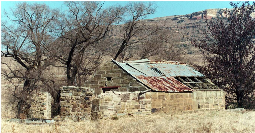
Fig. 129 Mill from the north (2000)
