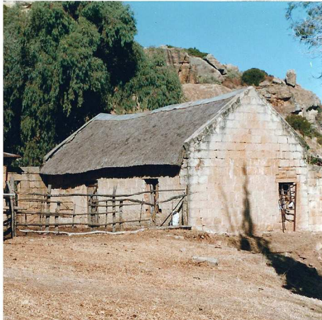
Fig. 176 North-eastern corner of house (1999)
