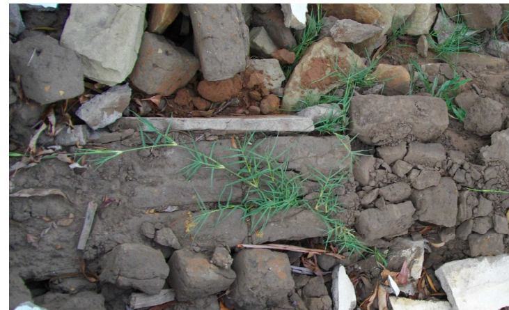
Fig. 274 House Grobler (a blacksmith's house) on Brindisi, the Middleton Estate, where the sun-dried bricks of an interior wall became visible after the house was demolished recently. (Photo: Louis du Preez 2012)
