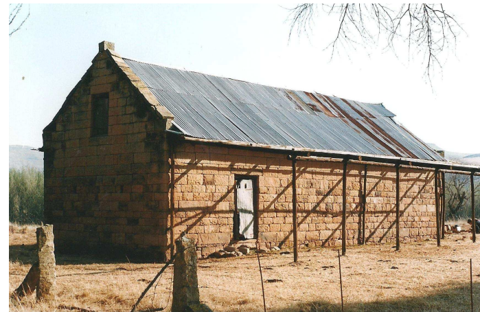
Fig 281 The shed behind Tierhoek House Fourie with different course heights and less careful jointing when compared to the house. (1999)
