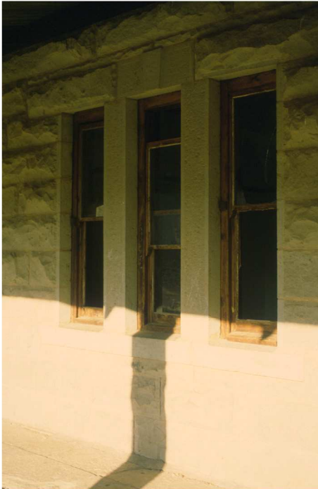
Fig. 73 Detail of windows on Lusthof stoep showing a lintel over the central window with punched finish and raised pseudo keystone. (1999)
