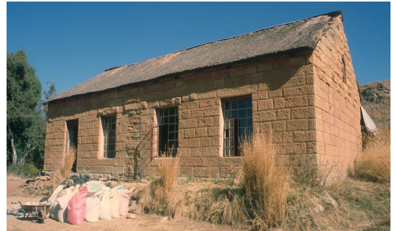
Fig. 92 Front of School Building facing east (1999)
