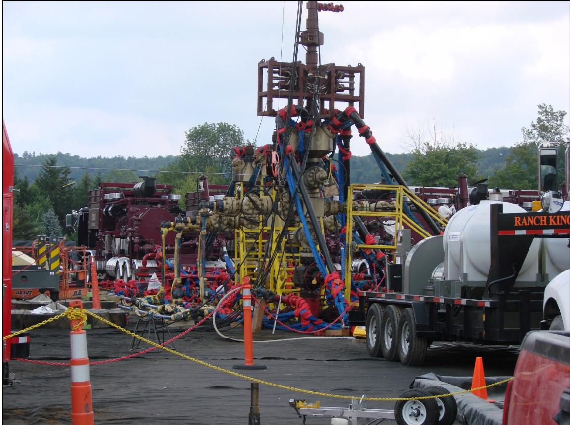
Figure 36: Well pad liner to prevent any contamination from surface spills (courtesy of D. Vermeulen, 2011)
