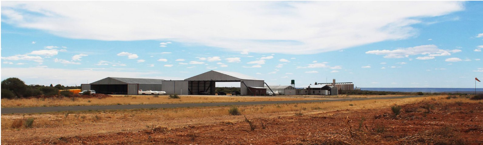
Photograph of existing hangars on site. Photograph by H.F. van den Berg. 2019
