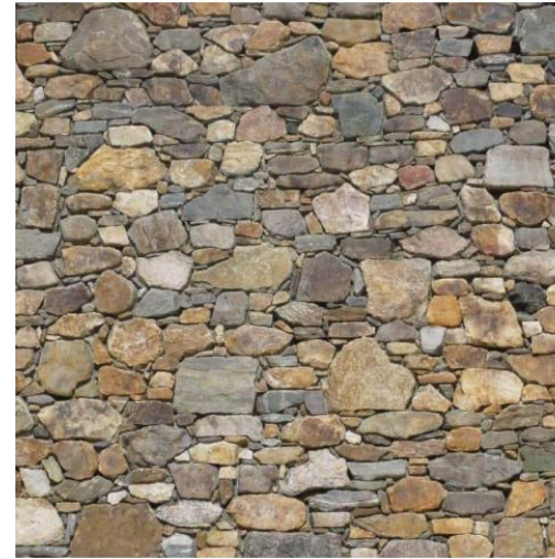
Image of uncoursed stone masonry. (source: https://gharpedia.com/ )
