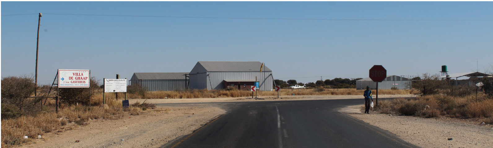
Photograph of site when approaching Douglas from Kimberly. Photograph by H.F. van den Berg. 2019
