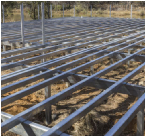
Image of lightweight galvanized steel support structure. (source: https://www.eva-last.co.za/ )
