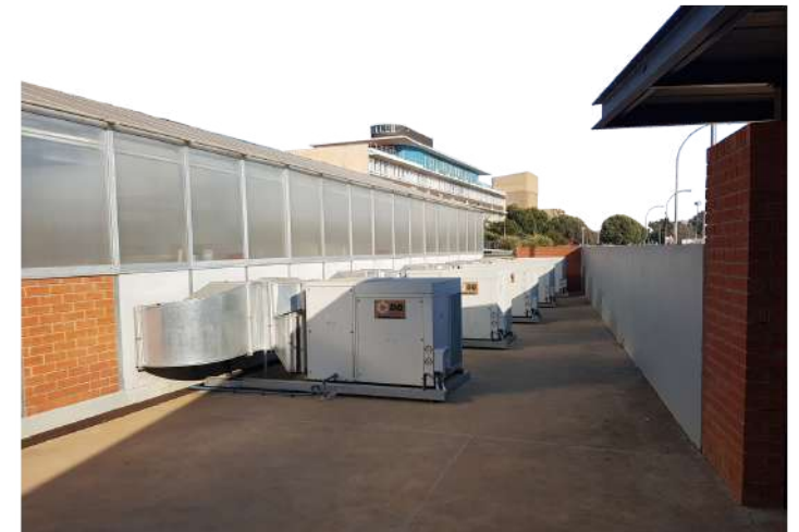
Figure 67 - Greenhouse exterior illustrating approx 1800mm brick wall with HVAC penetrating into interior space (Du Preez, 2021).
