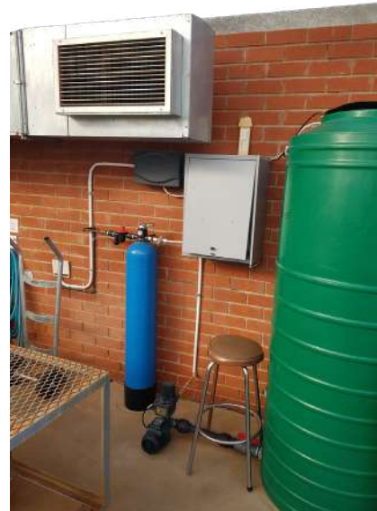
Figure 63 - JOJO tank, compressor and water filter mounted on wall (Du Preez, 2021).
