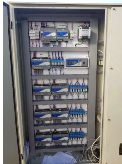
Figure 66 - Climate control panels on the exterior of greenhouse (Du Preez, 2021).
