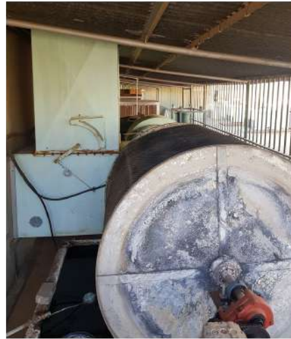
Figure 59 - Evaporative cooling system on building exterior (Du Preez, 2021).
