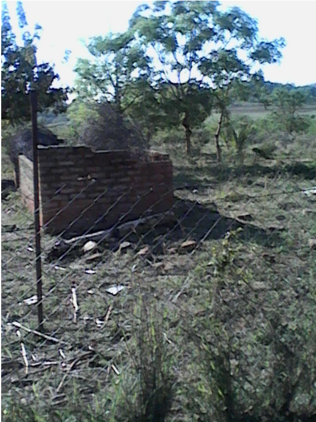
Plate 4.6: Untreated wooden posts prone to termites attack and susceptible to elements of weather (Chinyamatumba)
