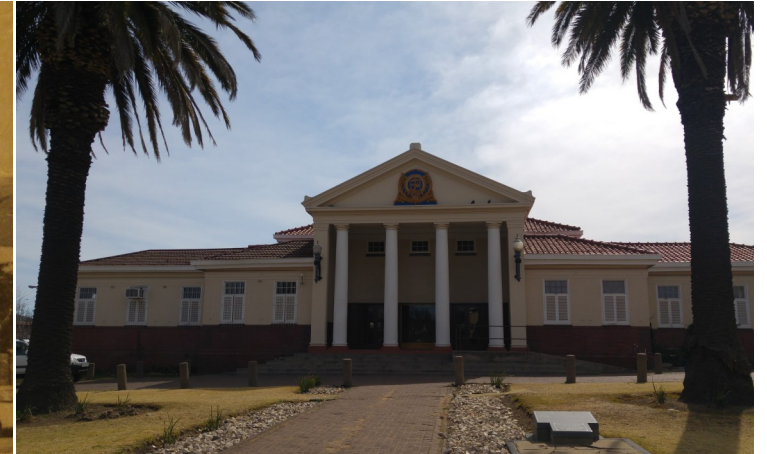
Fig 45.The Town Hall, built in 1829. . (Scholtz,1976: 59)
