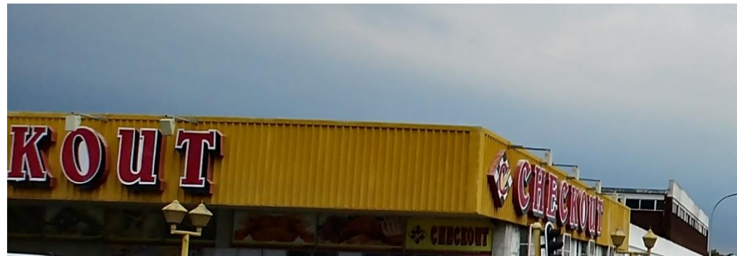
Fig. 40.b. Top image of the Checkout Store roof.
