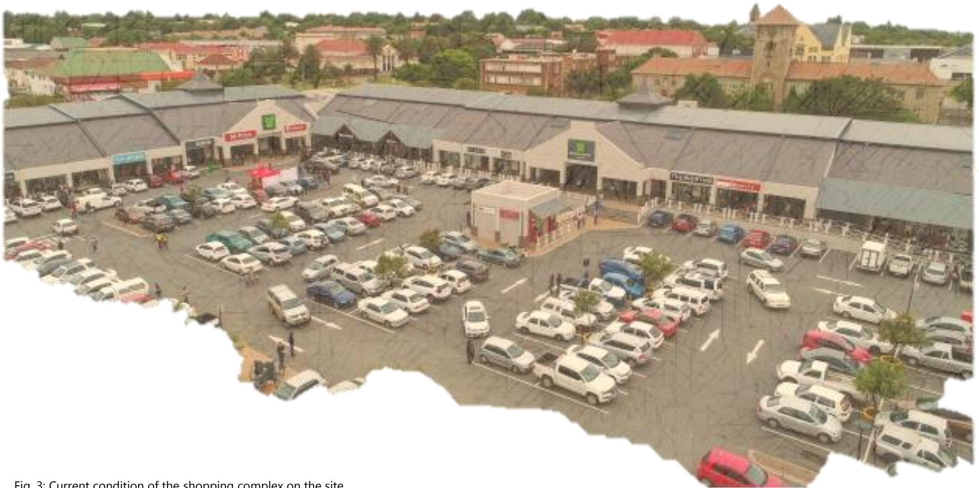
Fig. 3: Current condition of the shopping complex on the site
