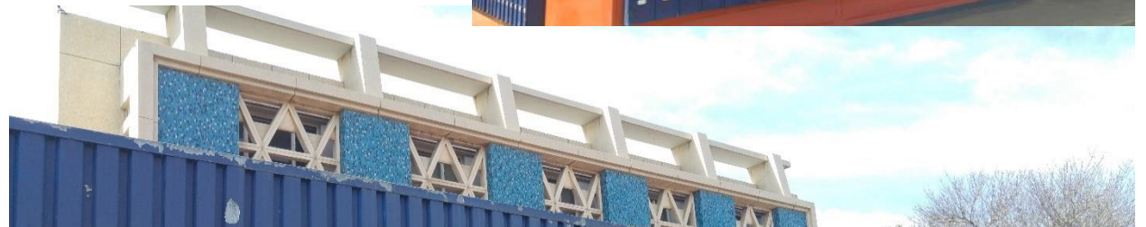
Fig. 40.d. The top of the western façade of the Standerton Post Office.
