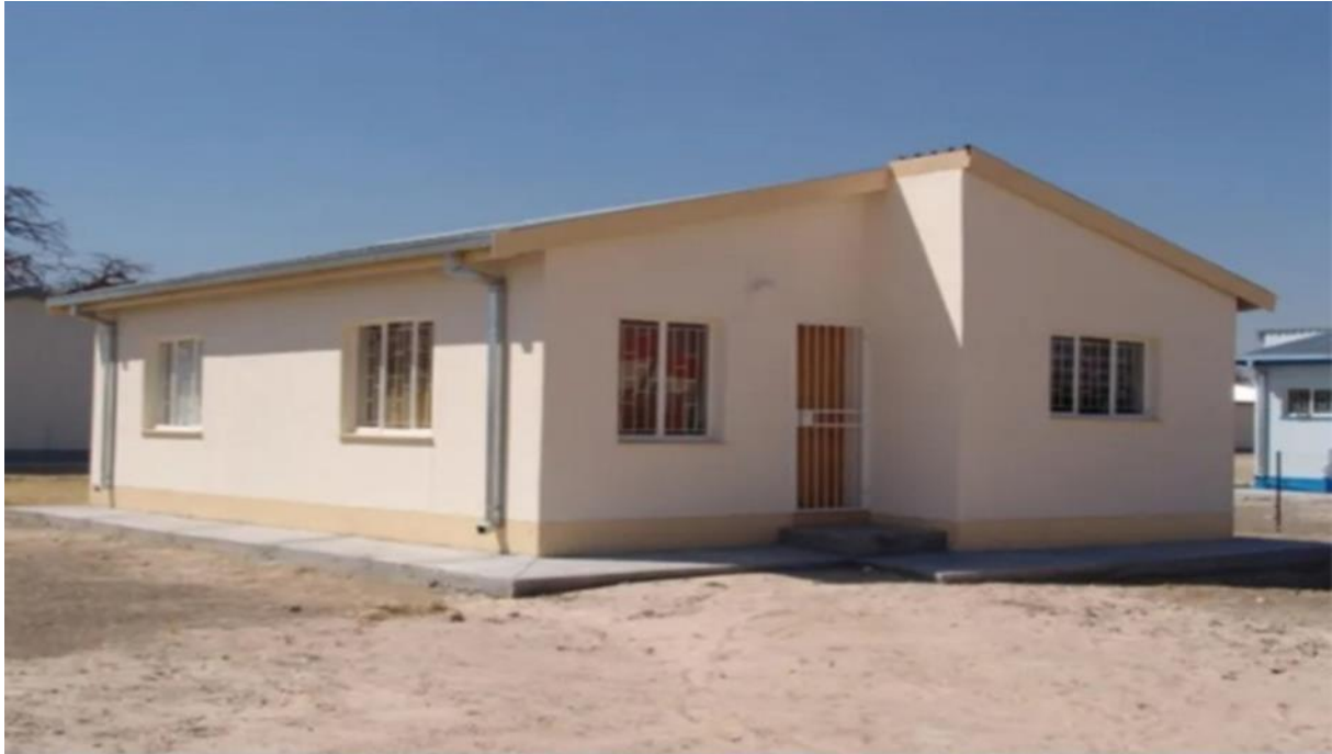
Figure 2.3 NHE house in Omuthiya town (Source: Matheus)
