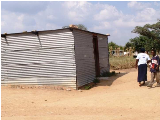
Photograph 4.18 The informal structure in Vingerkraal
