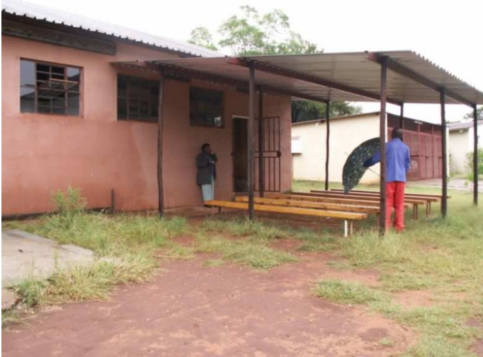
Photograph 4.8 The front view of the building at Phokeng Clinic
