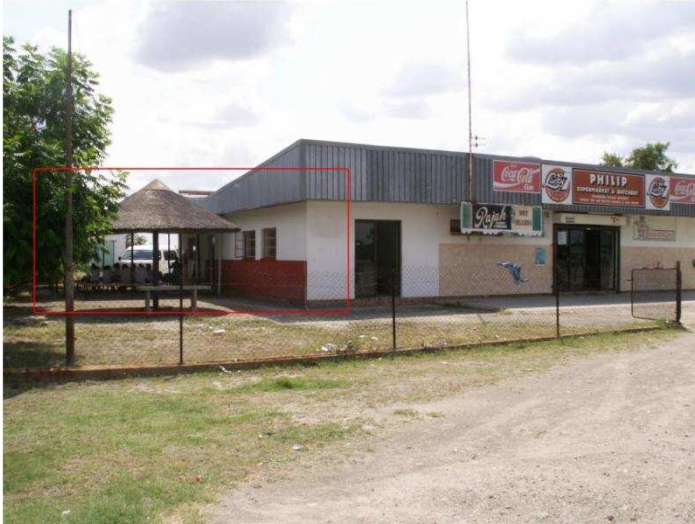
Photograph 4.10 The building that houses the Tlaseng Clinic
