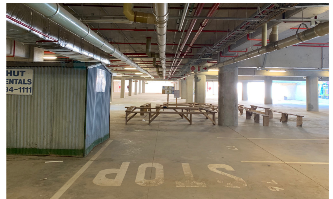
Figure 4.99 Javett Art Centre at UP basement (Author, 2019)
