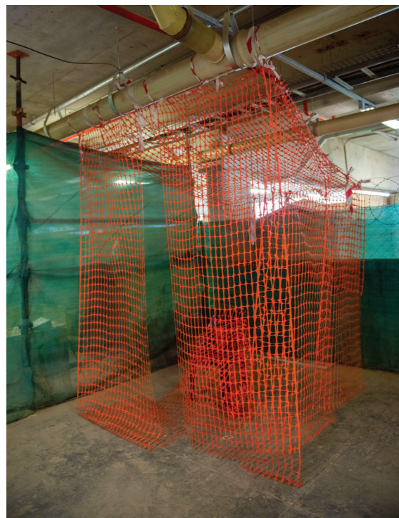
Figure 4.108 Safety net house installation (Pretorius, A. 2018)
