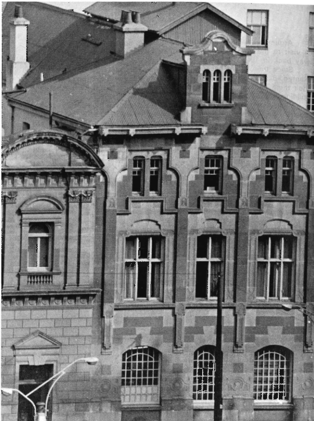
Figure 5.122 Annex of the National Bank and Mint (photograph by Pretoria News, December 1975).
