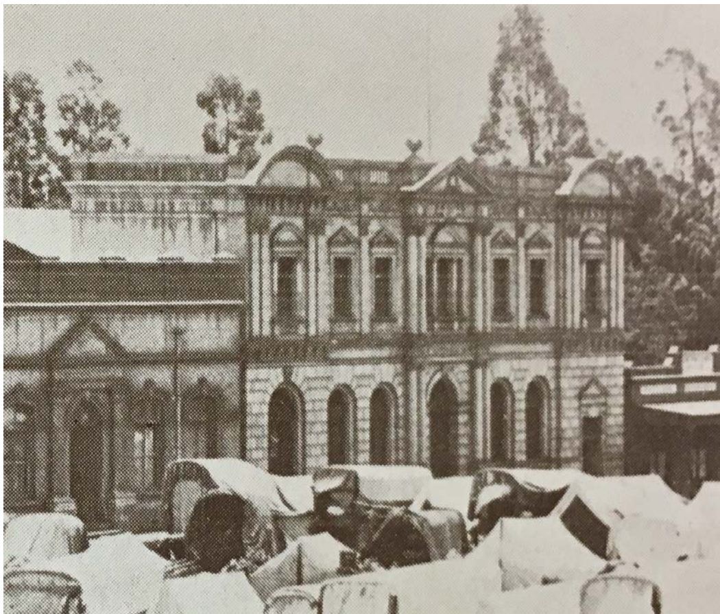
Figure 5.116 The National Bank and Mint with Kimberley Hotel to the right and Post Office to the left, photograph taken during Nachtmaal around 1897 (Dunston 1975: 33).
