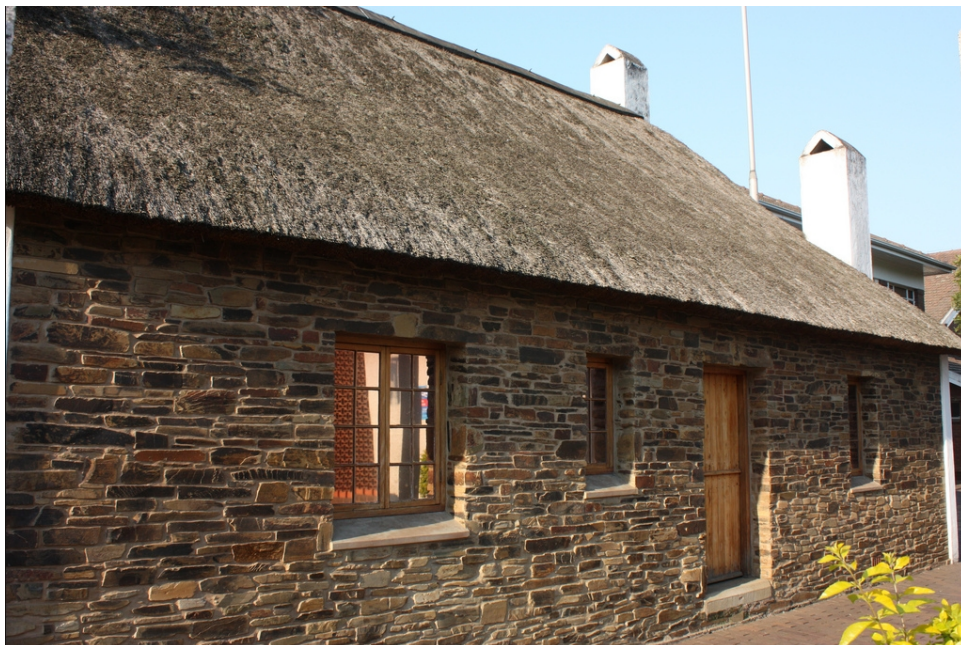
Figure 5.50 Andries Pretorius's house on Welverdiend, near Pietermaritzburg was rebuilt 11km from its original location (retrieved from http://boereafrikana.com/Mense/Groot_Trek_Leiers/Andries%20Pretorius/apretorius_huis.jpg ).
