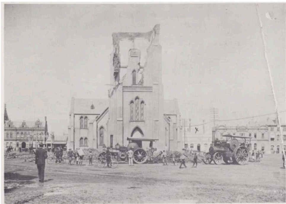
Figure 5.15 Traction engines attempted to pull down the tower of the second church in 1905 (Allen 1971: 34).
