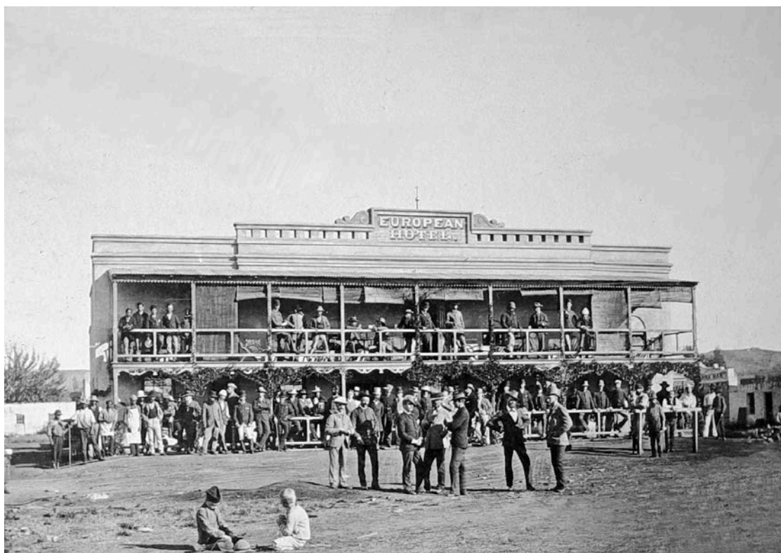
Figure 5.40 European hotel after it was rebuilt in 1880 (retrieved from the public domain: https://web.facebook.com/photo.php?fbid=10210960482870392&set=pb.1303334893.-2207520000.1522136213.&type=3&theater ).
