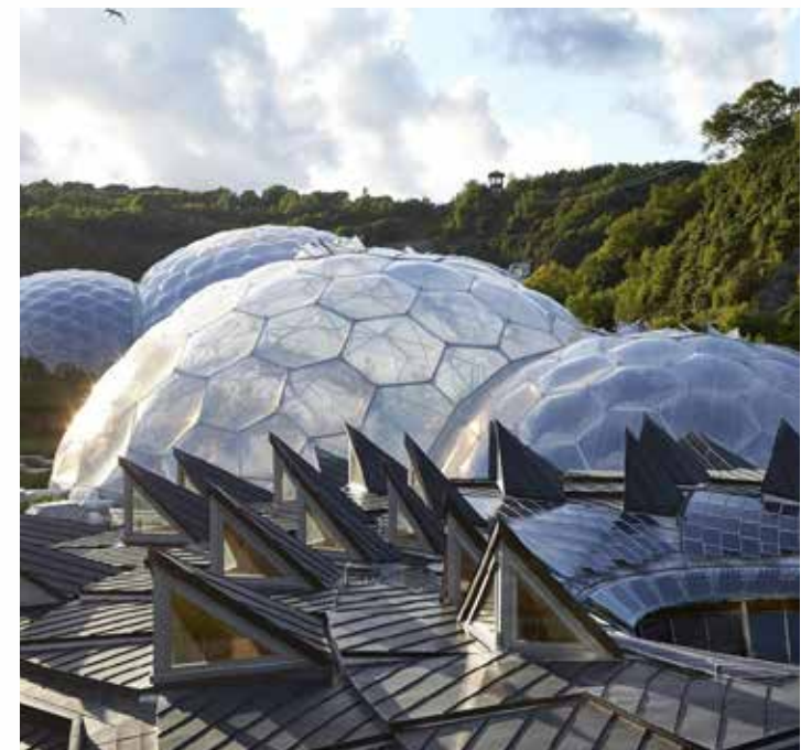
Figure 174, Solar panels core roof (Grimshaw Architects, 2023: online)
