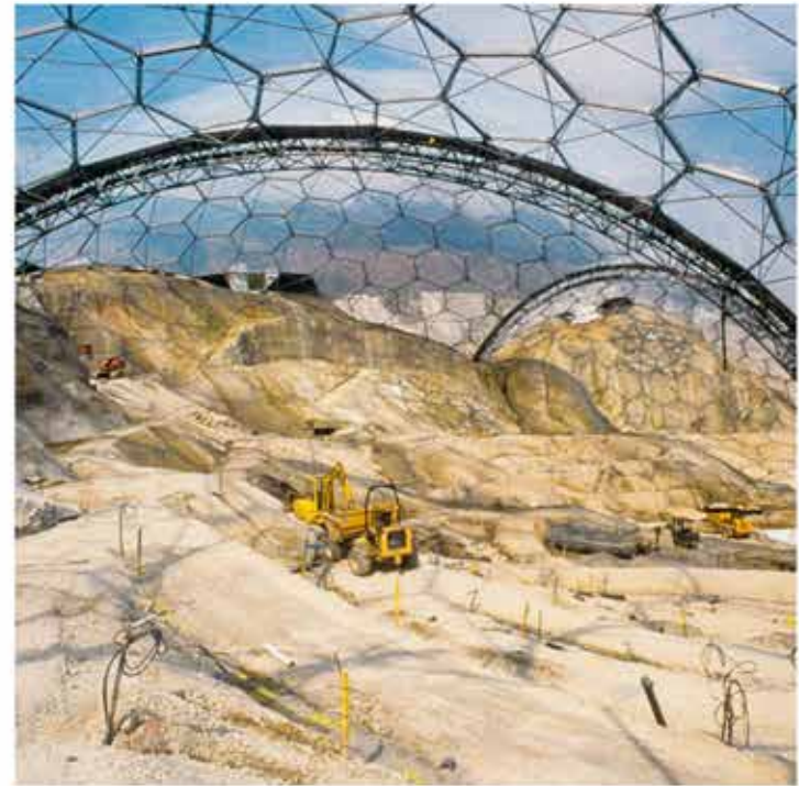
Figure 171 Before planting (Grimshaw Architects, 2023: online)
