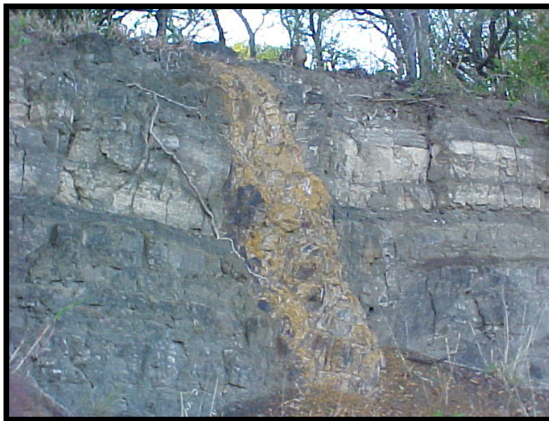
Figure 2.14. Roots directed to the nutritious, weathered and fractured diabase intrusion in contrast with the almost absent roots in the shale of the Mozaan Group. The intrusion supports different tree species to those encountered on the shale plains. Note the deformation of the shale alongside the intrusion. Ithala Nature Reserve, Louwsburg, Kwazulu-Natal.
