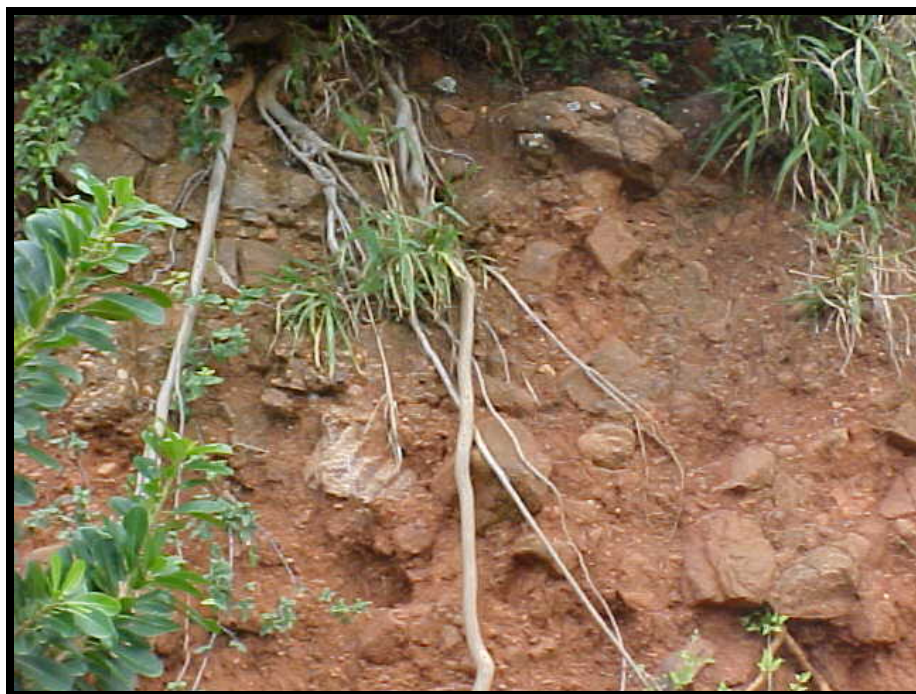
Figure 4.39. Conspicuous rooting of Ficus ingens along the fault zone.
