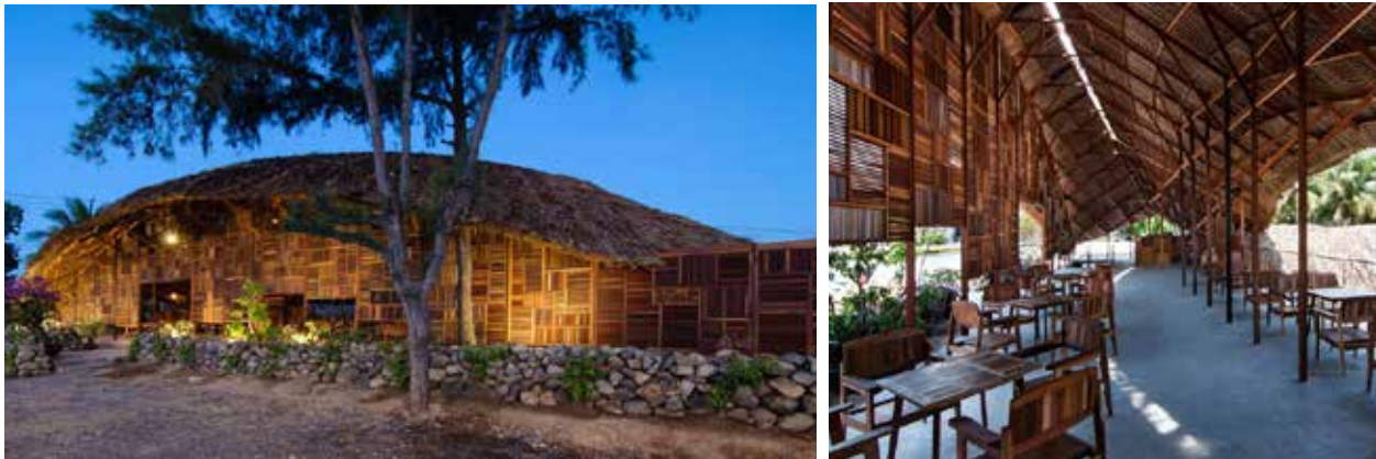
Figure 143 (left): Salvaged Ring Cafe, in Vitenam. Figure 144 (right): Interior view, revealing natural use of timber construction and a weaved grass ceiling and shading devices (A21 Studio, 2019: photos).
