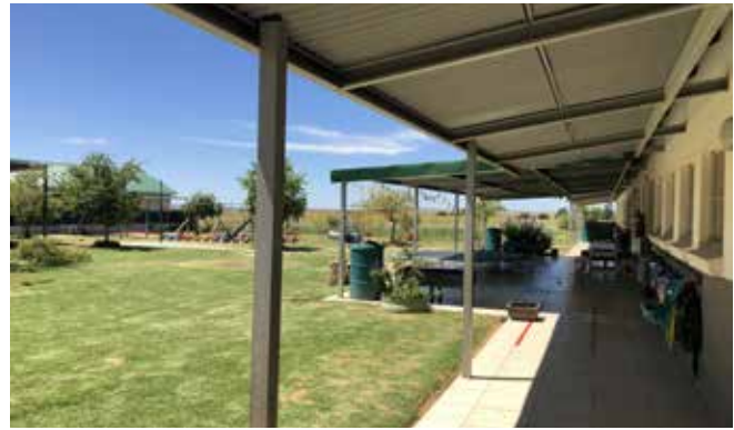
Figure 250: Existing Tjhabelang Primary School structure (Caldeira, 2019: photo).
