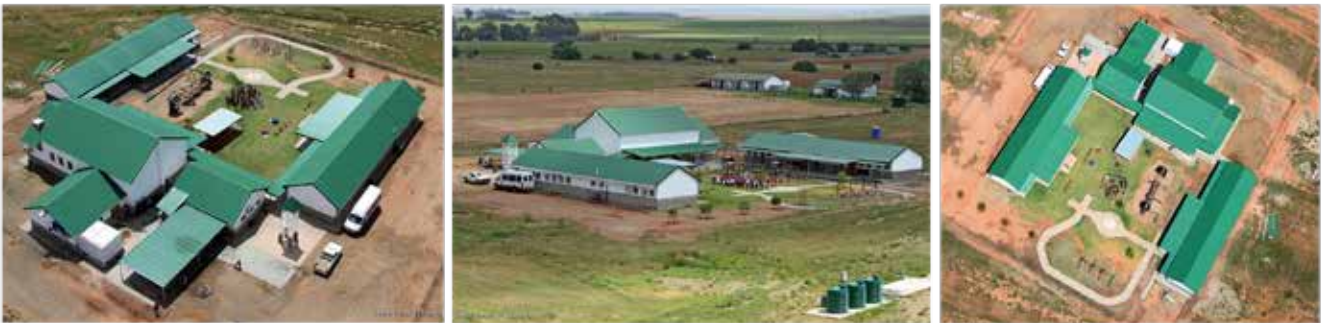
Figure 91, 92 and 93: Tjhabelang Primary School just after construction completion (Marais, 2010: photos).
