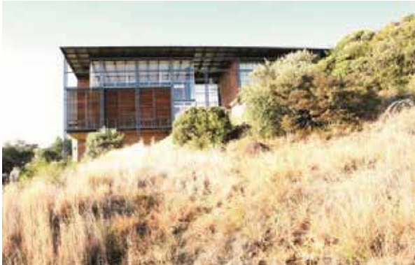
Figure 26 and 27: House Enkalweni in Bloemfontein, showing typical appearance of light steel structure with brick infill (Smit, 2019: photos).
