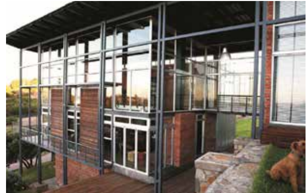
Figure 26 and 27: House Enkalweni in Bloemfontein, showing typical appearance of light steel structure with brick infill (Smit, 2019: photos).
