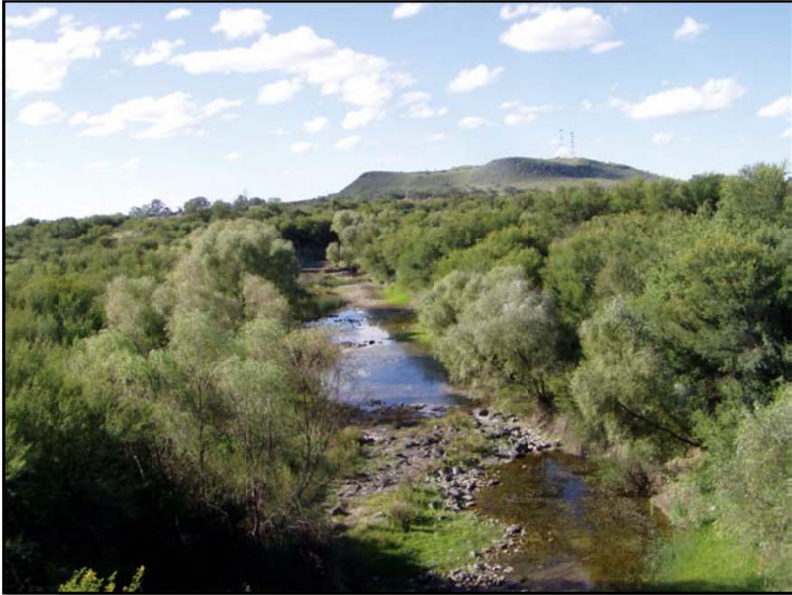
Figure 98: Vegetation cover stabilizes the banks of the Krugersdrift (Tsokeli, 2005)
