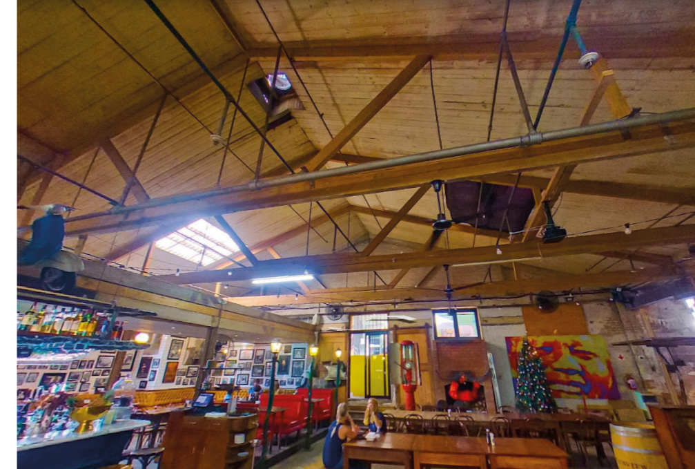
Figure 36: Timber trusses of older warehouses on site (Earth, 2023: online)
