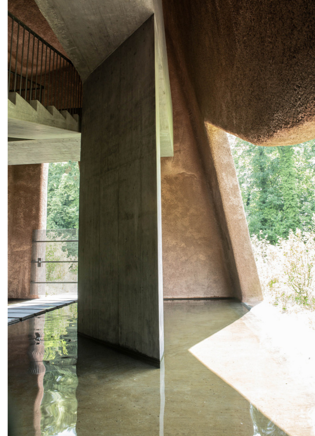
Figure 52: Photograph showing water covered floor at the entrance (Müller, 2017)
