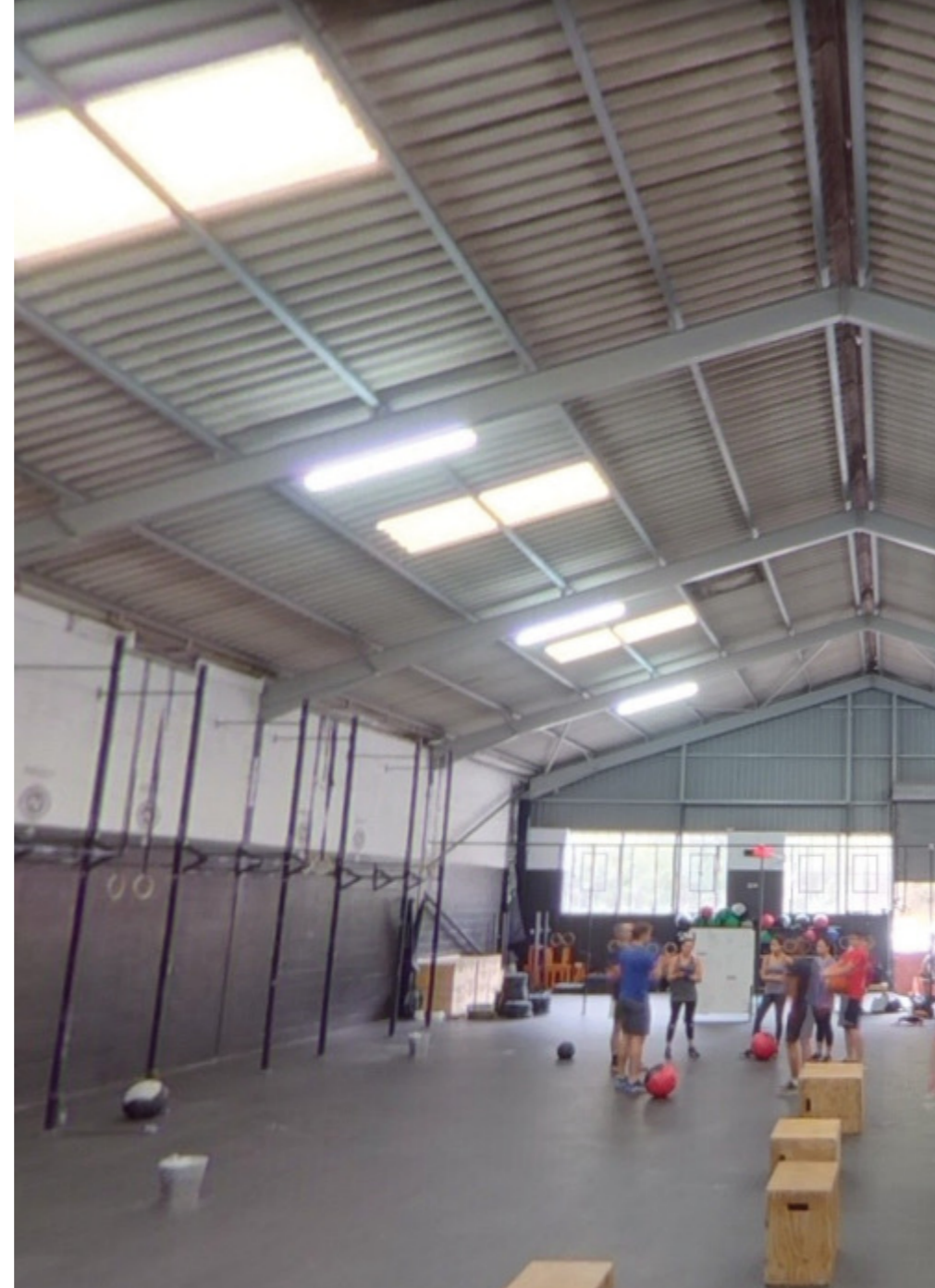
Figure 35: Steel construction of newer warehouses on site (Earth, 2023: online)
