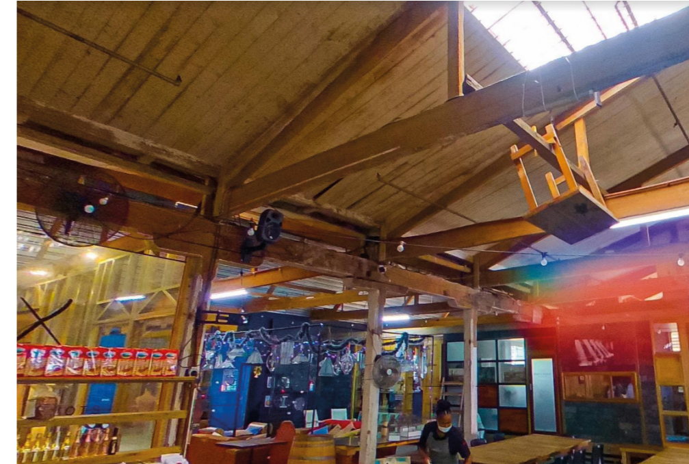
Figure 37: Timber columns and beams of older warehouses on site (Earth, 2023: online)
