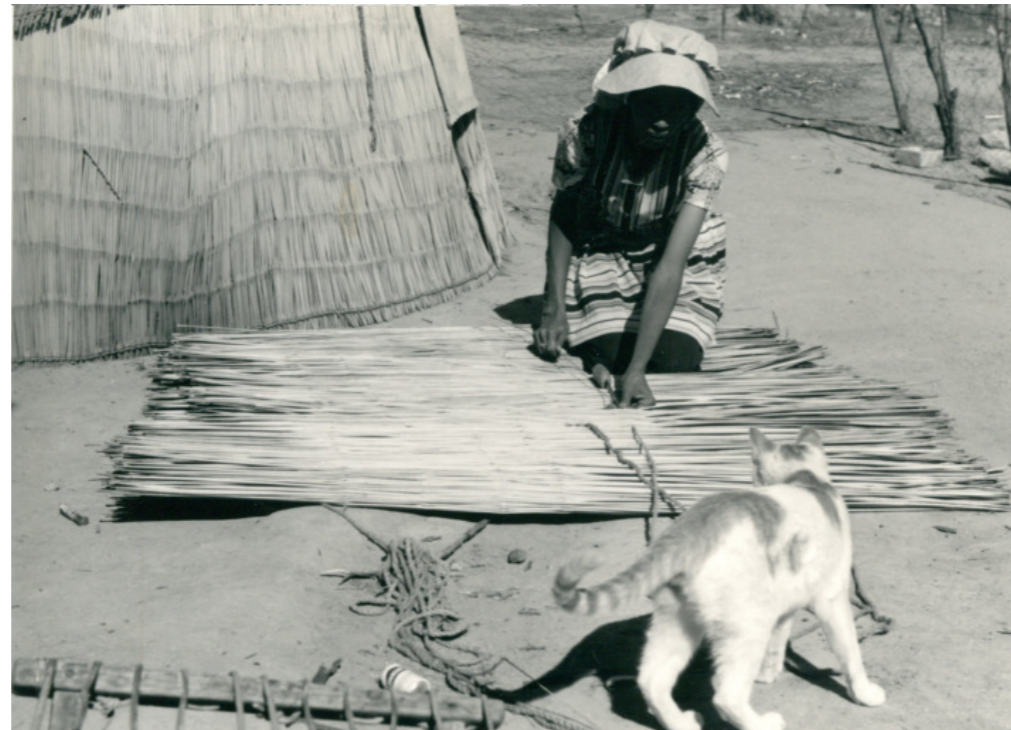
Figure 33: Weaving reeds with hessian rope (Walton, 1978)
