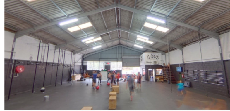
New Warehouses (Steel construction)
