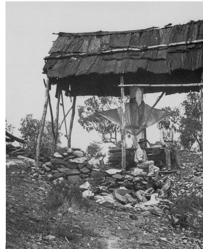
Figure 37. Some miners from the Broken Hill mine standing beside an opening to a mineshaft where they had rigged some canvas to catch the wind and scoop fresh air down into the tunnels, resembling a system of wind-aided evaporation (Bleuscape Design, 2014: online)
