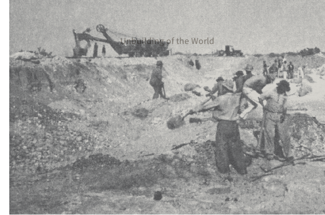
Figure 45. Down to Bedrock, 1950 - workers at bedrock level (Carstens, 2001: 92)
