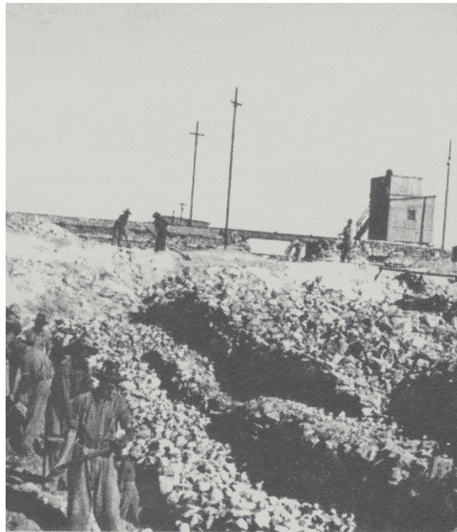
Figure 24. Surveillance, 1930s - excavating near superintendent (Carstens, 2001: 91)
