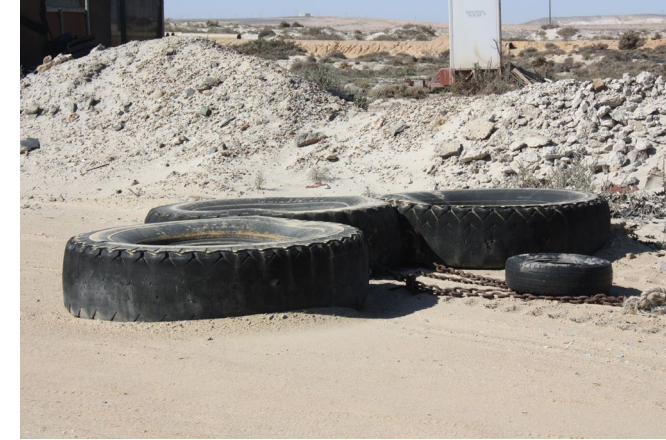
Figure 147. (right) Retaining Barrier - recorded on site (author, 2023)
