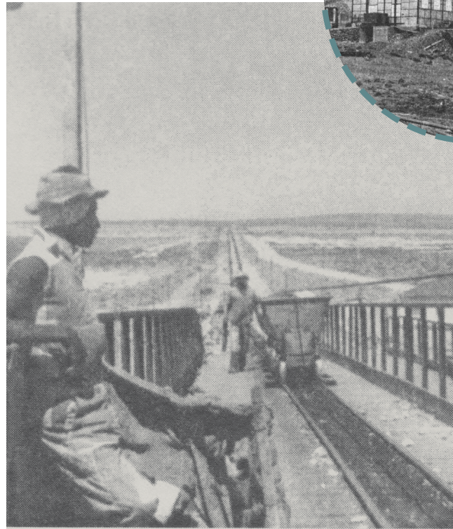
Figure 27. Owambo Trammers - trammers are shown on the ramp (Carstens, 2001: 90)
