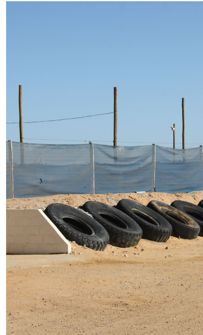
Figure 148. (above & left) Tire Walls - rammed earth encased in steel-belted rubber (recycled automobile tires) (Pangea Builders, n.d.: online)
