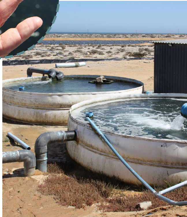
Figure 60. Ulva Baths 3 - Water reservoirs & filtration system with a pump house (author, 2023)
