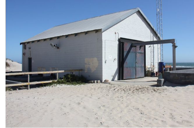
Figure 3. Pump House - existing infrastructure (author, 2023)
