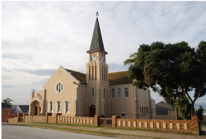
Figure 3.171: Photos of DRC Port Elizabeth after additions (2021)
