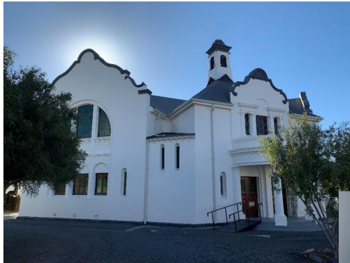
Figure 3.30: Photos of DRC Beaufort West church hall (2021)
