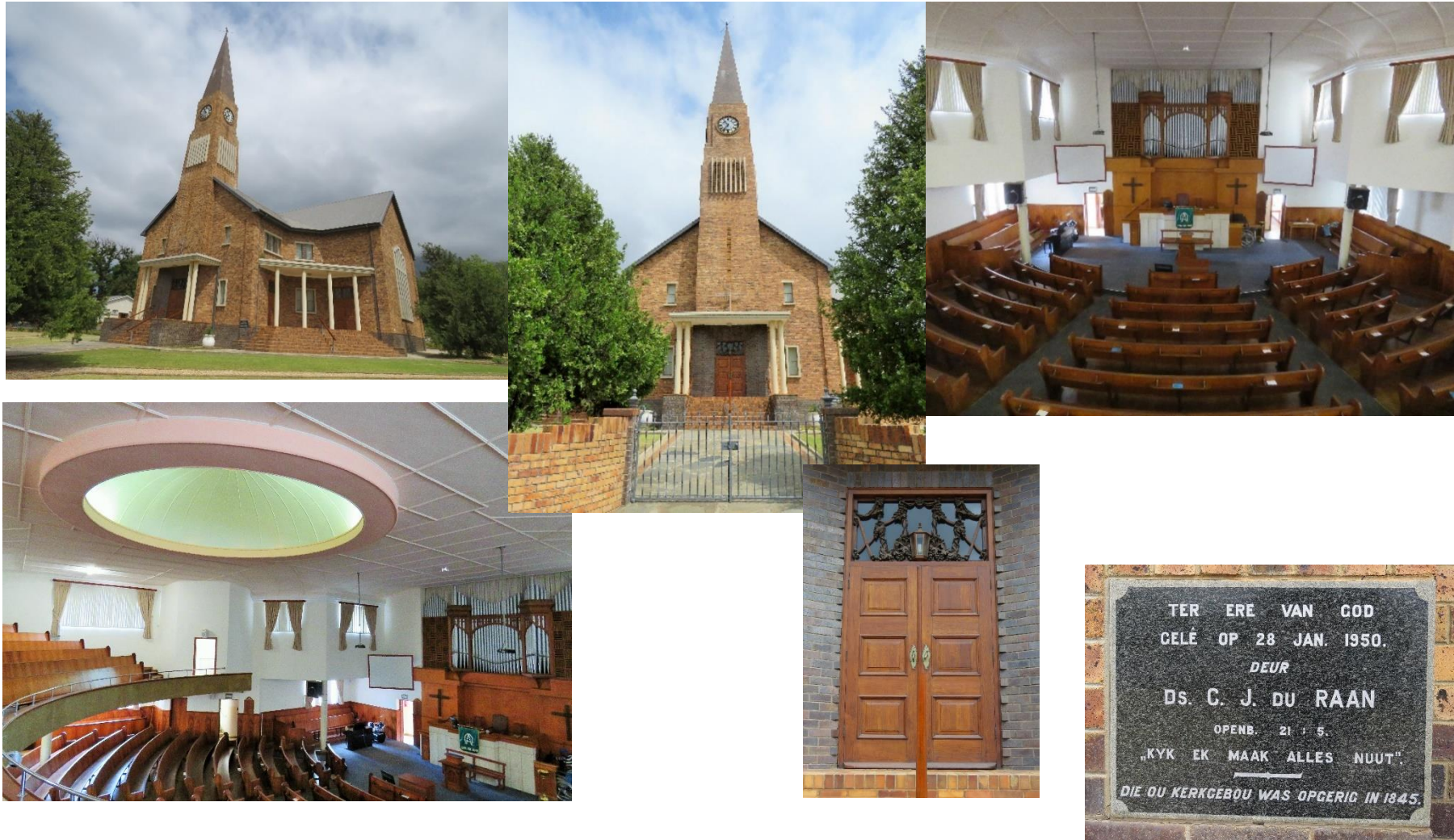
Figure 3.166: Photos of DRC Villiersdorp (2017)
