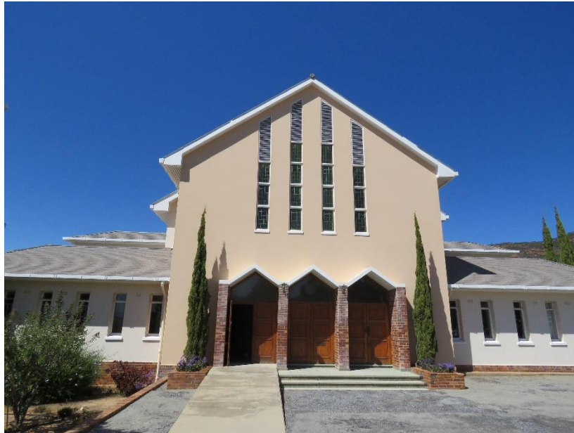
Figure 3.208: Photos of DRC Piketberg church hall (2017)
