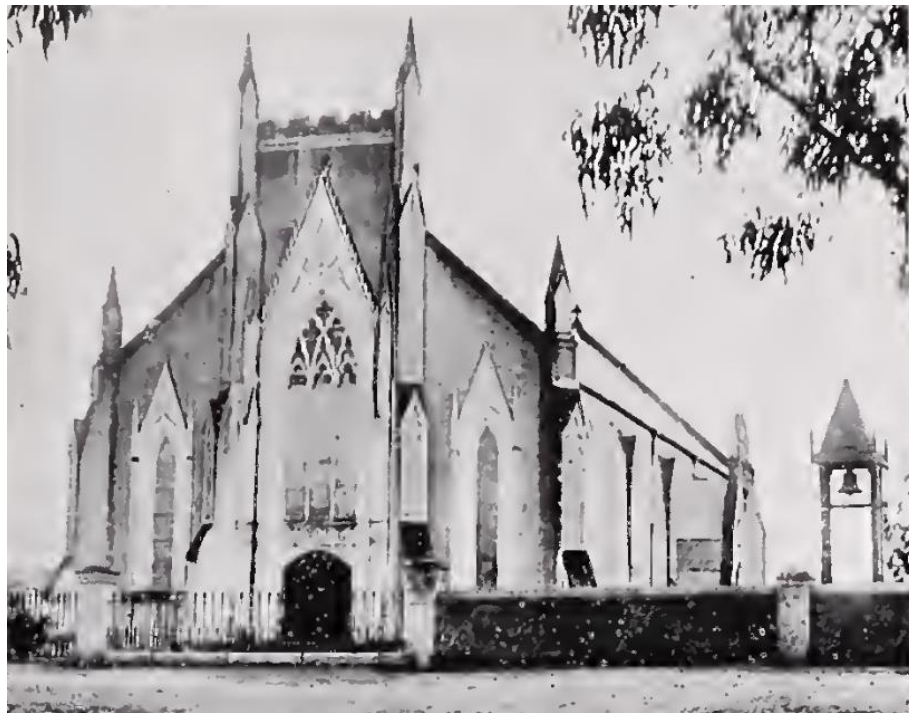
Figure 3.5: Photo of DRC Heidelberg, Cape, designed by CO Hager (Maeder & Zinn, 1917: 100)
