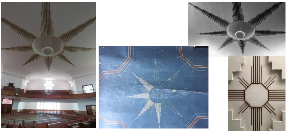
Figures 6.83, 6.84 and 6.85: DRC Somerset West: photos and plan of the art deco ceiling light (2017) and plan (DRC Somerset West church office)
