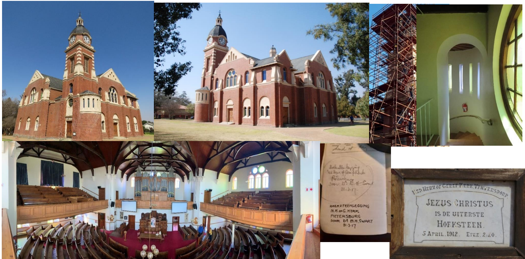
Figure 3.19: Photo of tower under repairs (DRC Ventersdorp church office)
