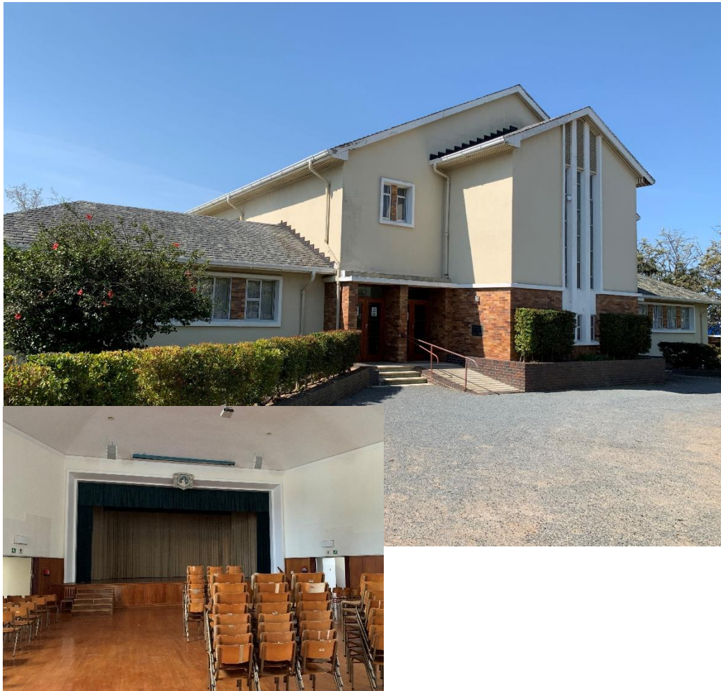
Figure 3.200: Photos of DRC Bredasdorp church hall (2021)
