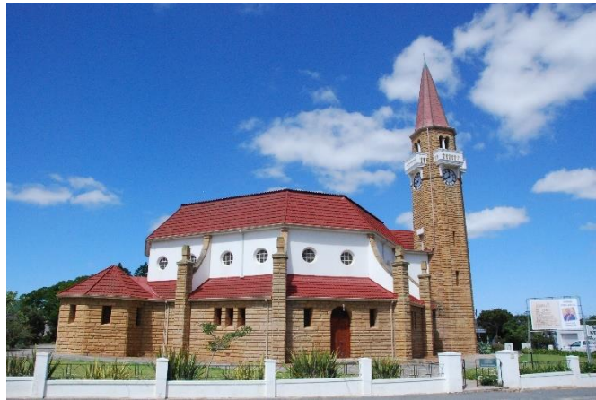
Figure 3.103: Photos of DRC Stanford (2021)
