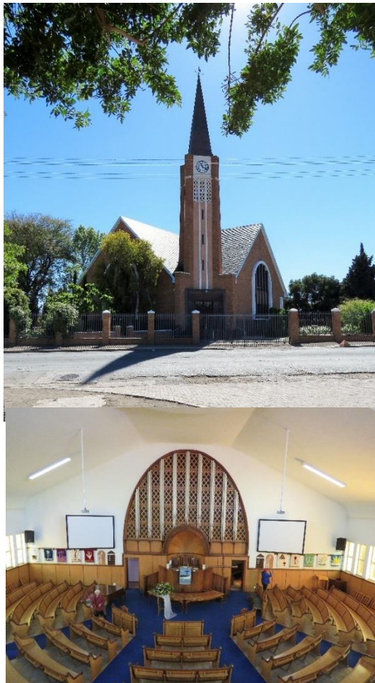
Figure 3.185: Photos of DRC Gamka East (2017)
