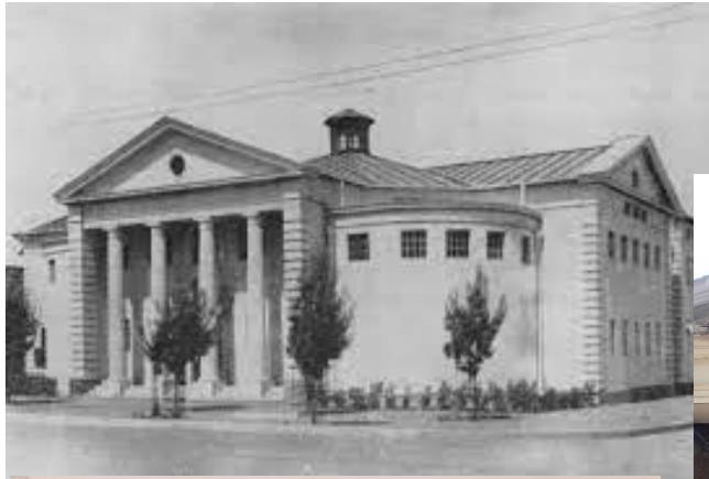
Figure 3.85: Photos of DRC Jubileum Hall (M Geldenhuys, 2022)
