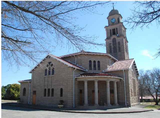
Figure 3.112: Photos of DRC Volksrust (2018)
