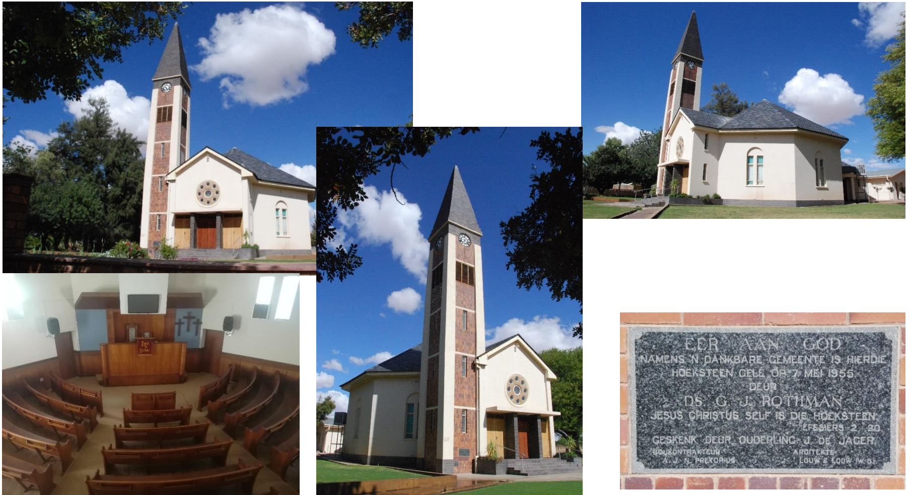
Figure 3.195: Photos of DRC Louisvale (2017)
