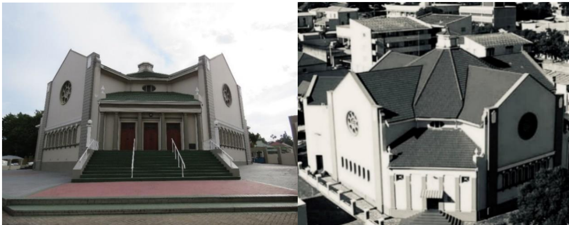
Figures 6.53 and 6.54: DRC Uitenhage: three entrance doors (2021) and an aerial view of the roof (Clive Botha, 2016)
