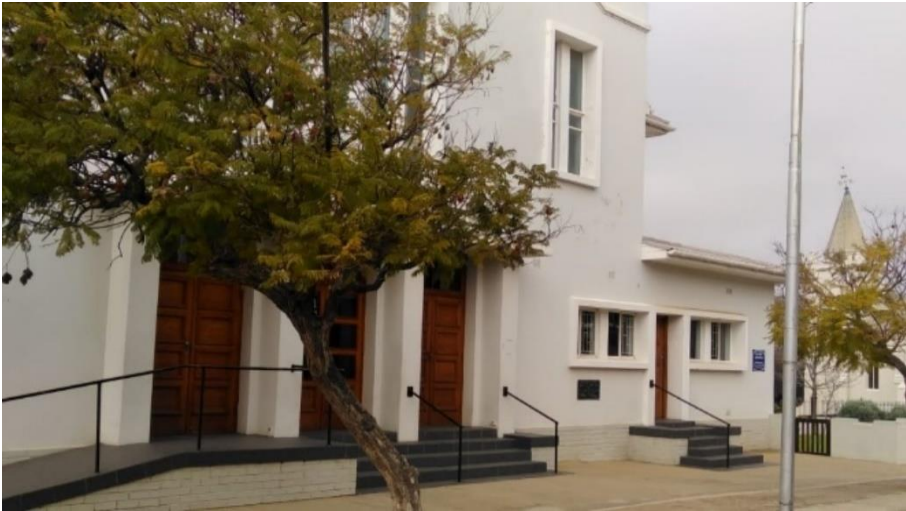
Figure 3.175: Photos of DRC Montague church hall (E Wright, 2022)
