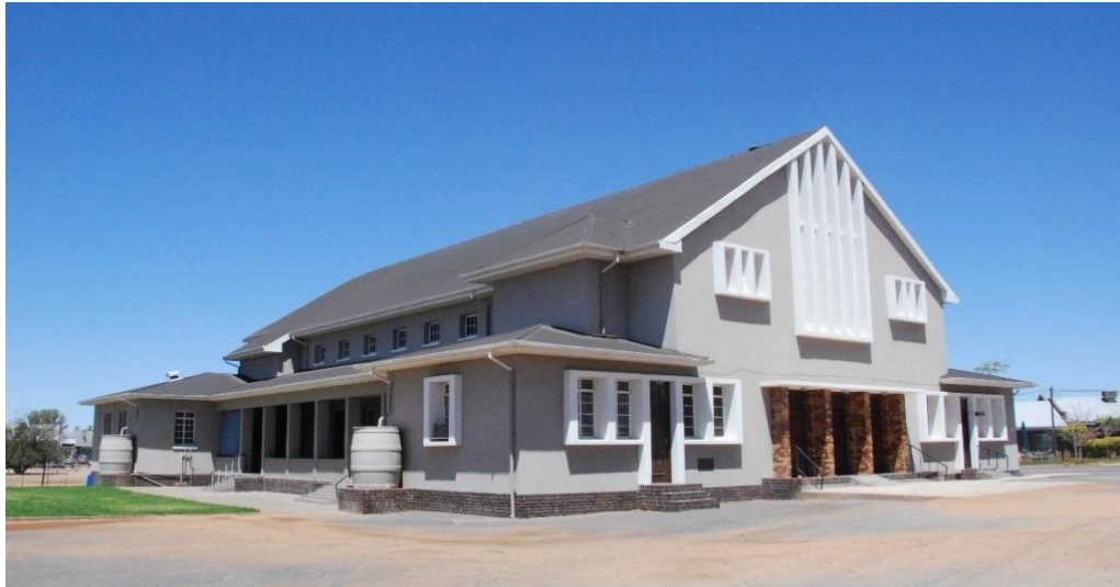
Figure 3.192: Photos of DRC Kakamas church hall (2017)
