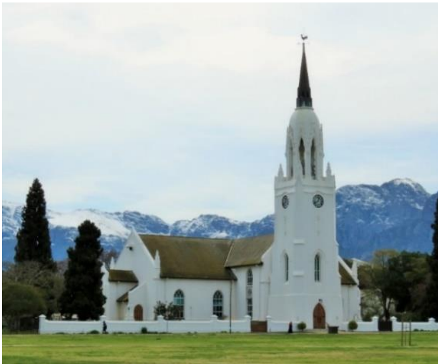
Figure 5.27: DRC Worcester with its tower designed by Wynand Louw (2021)
