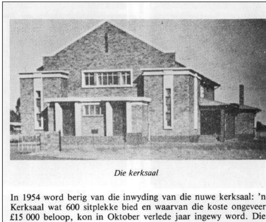
Figure 3.178: Photos of DRC Reivilo church hall (DRC Reivilo church office, 2019)
