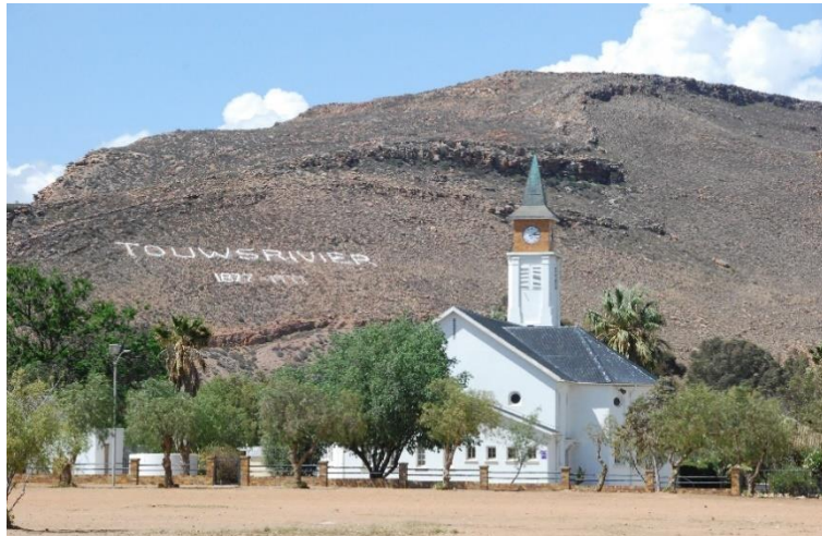
Figure 3.138: Photos of DRC Touws River (2017)
