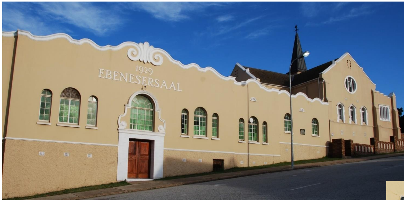
Figure 3.130: Photos of DRC Port Elizabeth Church Hall (2021)
