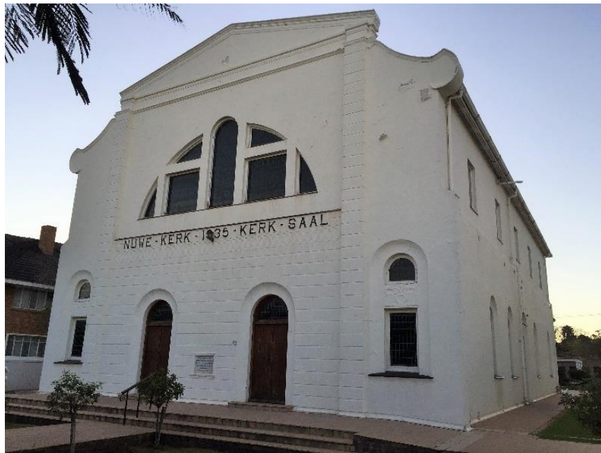
Figure 3.143: Photos of DRC Graaff-Reinet Nuwekerk Church Hall (2017 and top right - 2021)
