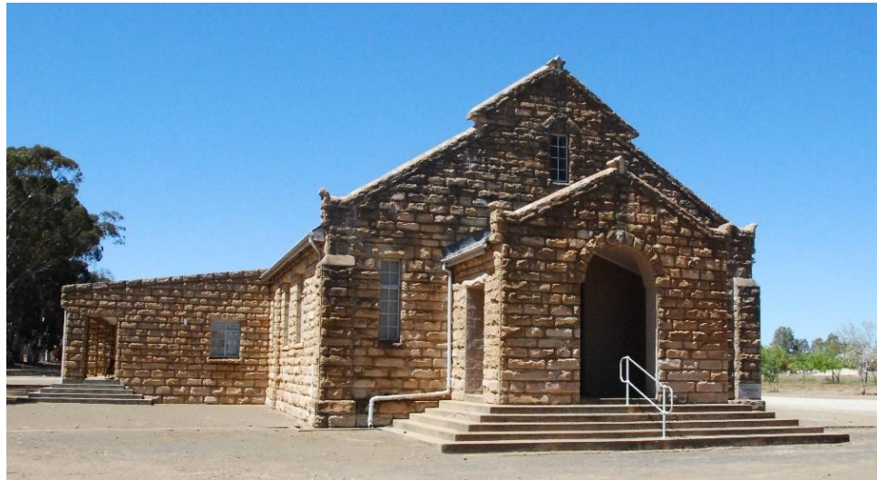
Figure 3.146: Photos of DRC Nieuwoudtville Church Hall (2017)
