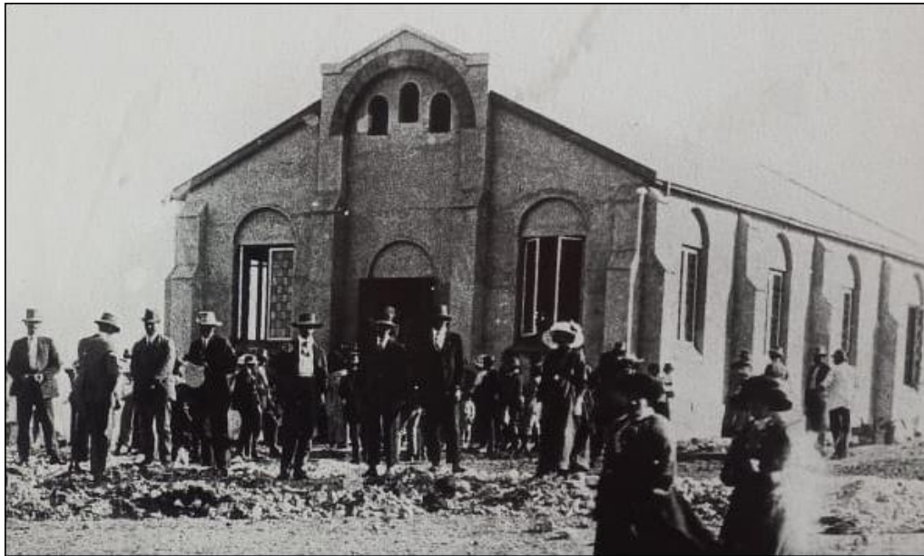
Figure 3.42: Photo of demolished DRC Deben (Van der Merwe, 2016: 35)
