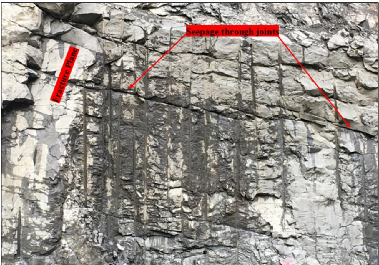
Figure 4-3 Central basalt zone, massive, with fractures, joints, and cracks from blasting.
