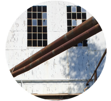
CORRUGATED IRON CLADDING
