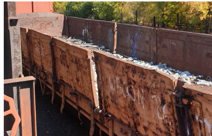
Fig. 05 Rusted elements on the site(Author,2019)
