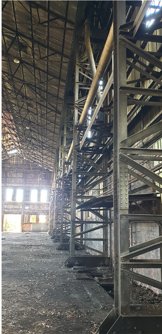
Fig. 13 The structure of the train terminal (Author,2019)
