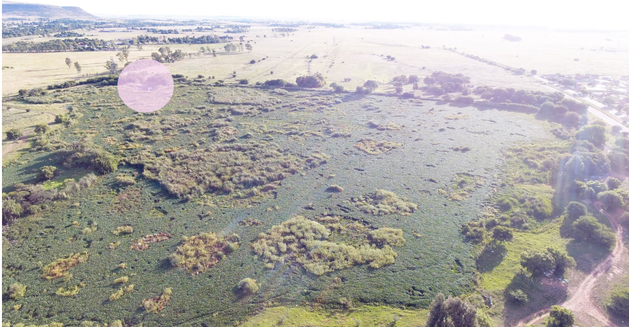
Figure 4: Illustration the overflow system on site (author,2023).
