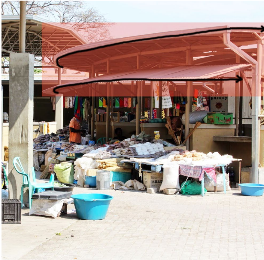
Figure 72: Illustrates double roof system (Pompert edited by author, 2023).
