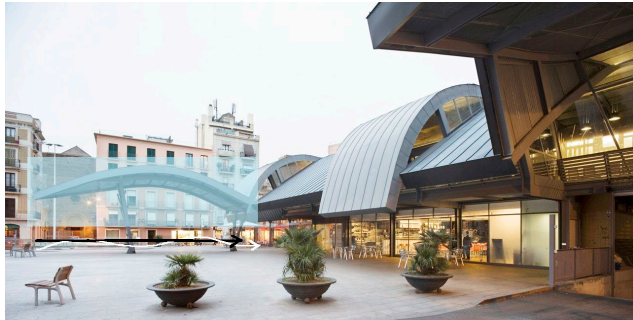
Figure 147: Roof structure, emphasising the entrance (Goula edited by author,2023).
