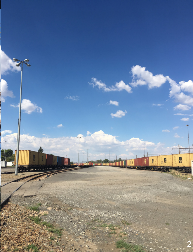
fig. 33 Railway depot towards North-east.
