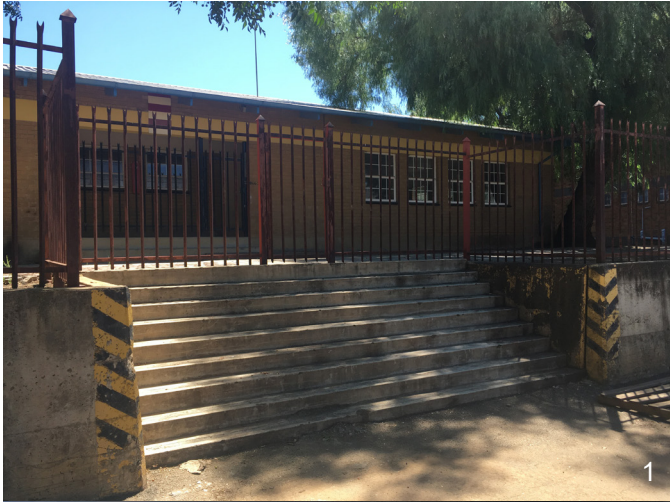
fig. 25 Existing stairs to admin building.
