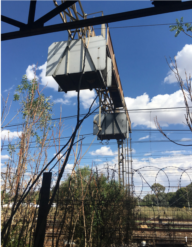
fig. 32 Railway view from site.
