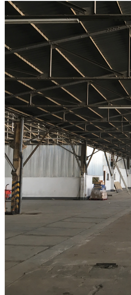
fig. 39 Interior view of existing s
