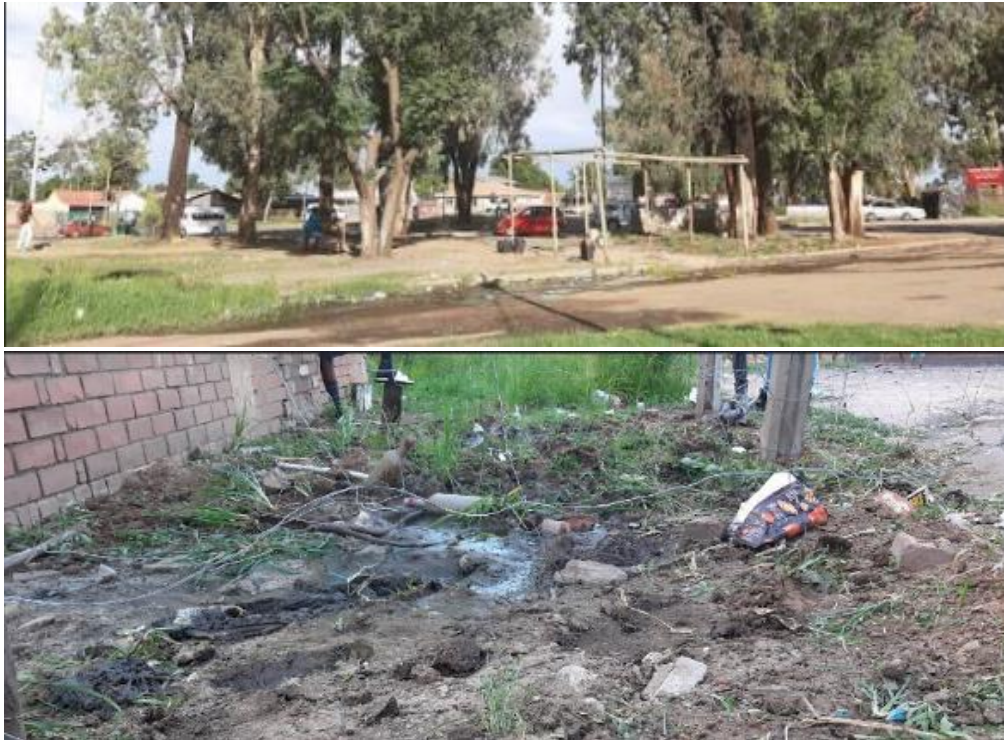
Figure 7.32: A View of Sewerage and Drainage Issues
