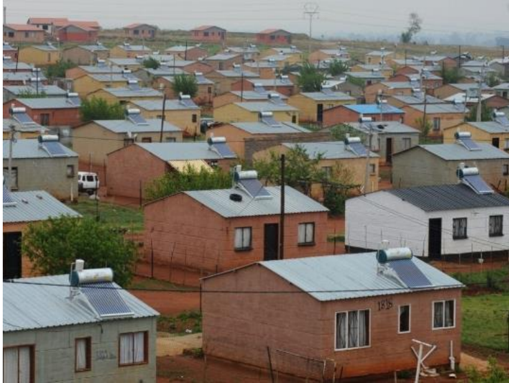
Figure 3.10: Township RDP Housing
