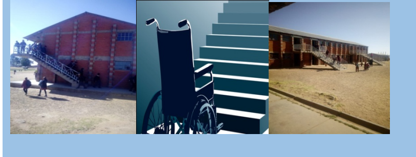
Figure: 4.4: shows that CwPDs have to climb the stairs to reach the classrooms
