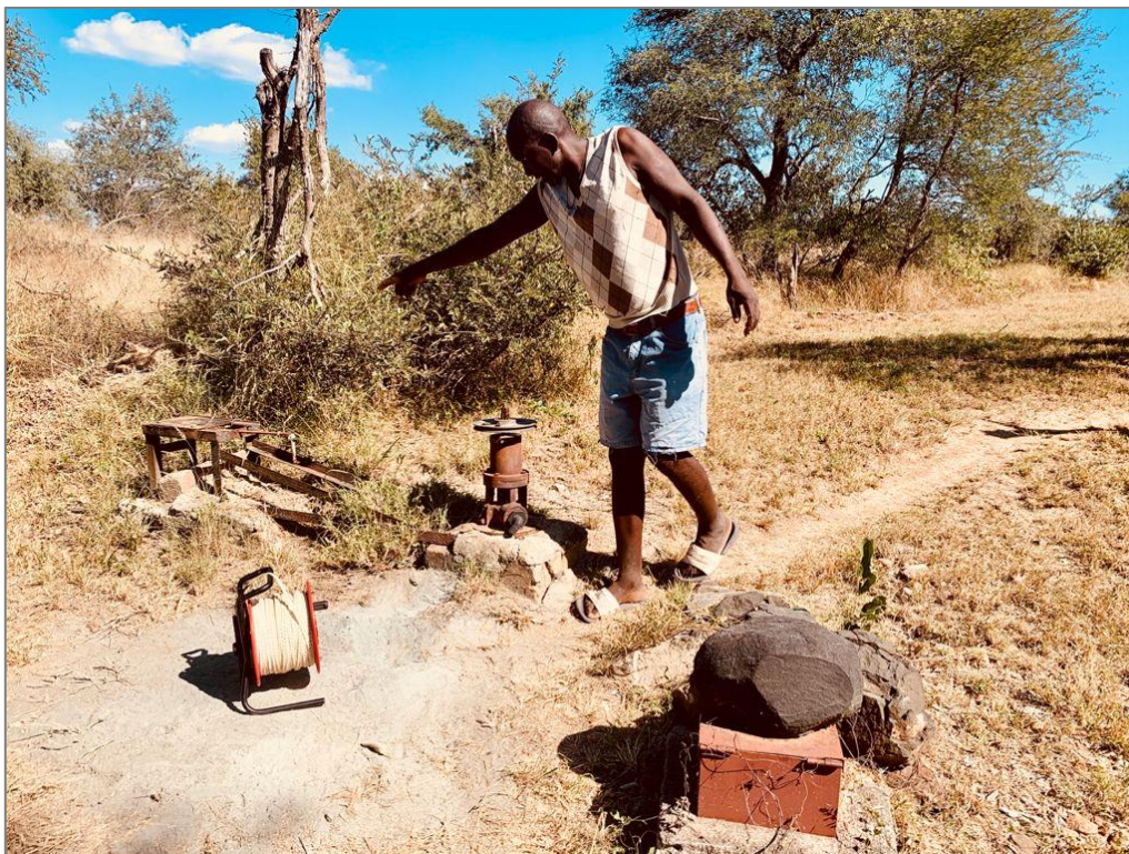
Figure 1 – Typical example of poor groundwater management. Three boreholes were drilled adjacent to one another over approximately 15 years.
