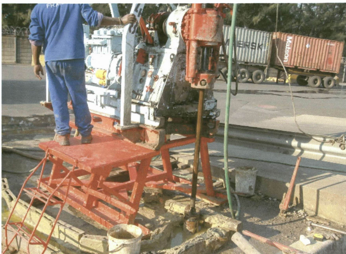
Figure 4.4: Rotary washbore drilling rig.
