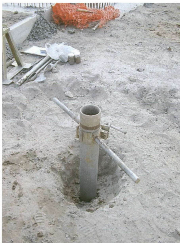
Figure 4.3: Hand auger hole with temporary casing.
