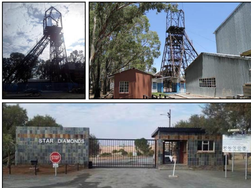
Figure 3.2: The Star Diamonds mine with shaft 4 that was used as the study site for this research.
