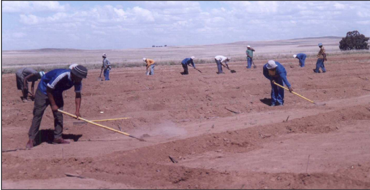
Figure 3.2 Workers busy preparing the IRWH system on communal scale.
