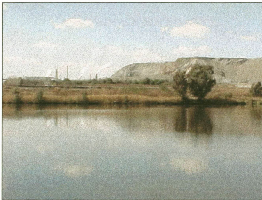
Figure 10: View from the earthdams at the waste disposal site, towards the SCI factory and coarse ash dumps.
