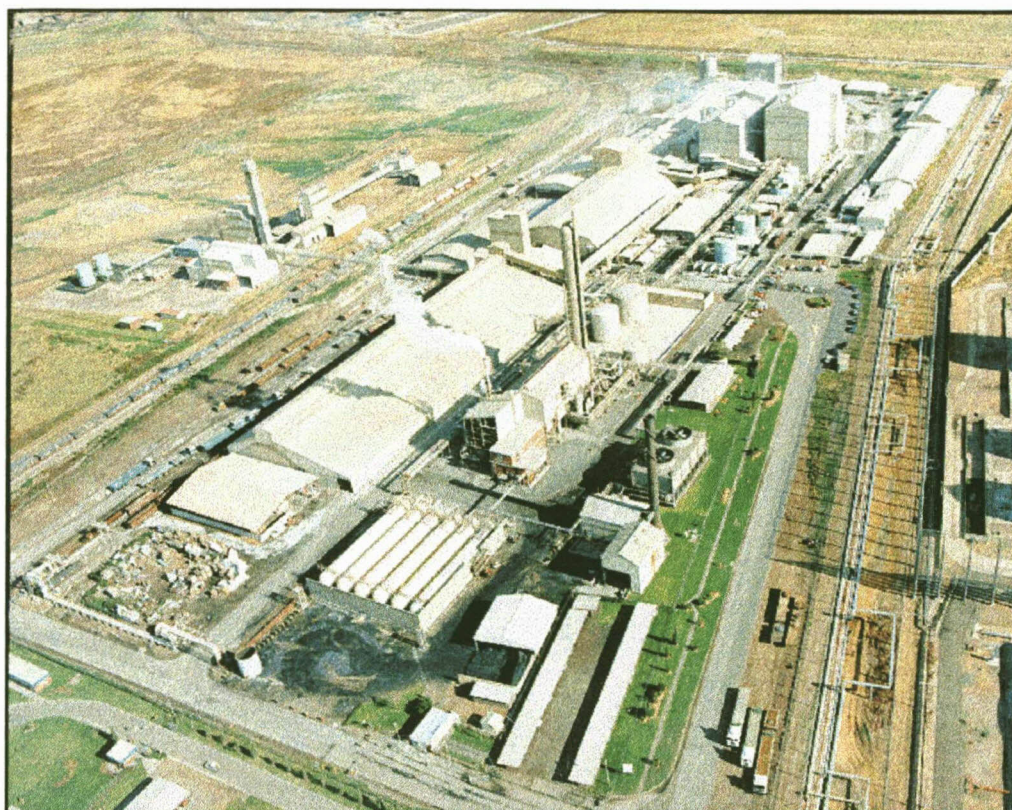
Figure 6: Omnia Fertiliser factory (Photo: Omnia, 1999)
