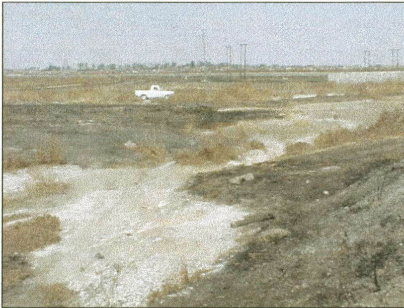
Figure 28: Venco Park Disposal area
