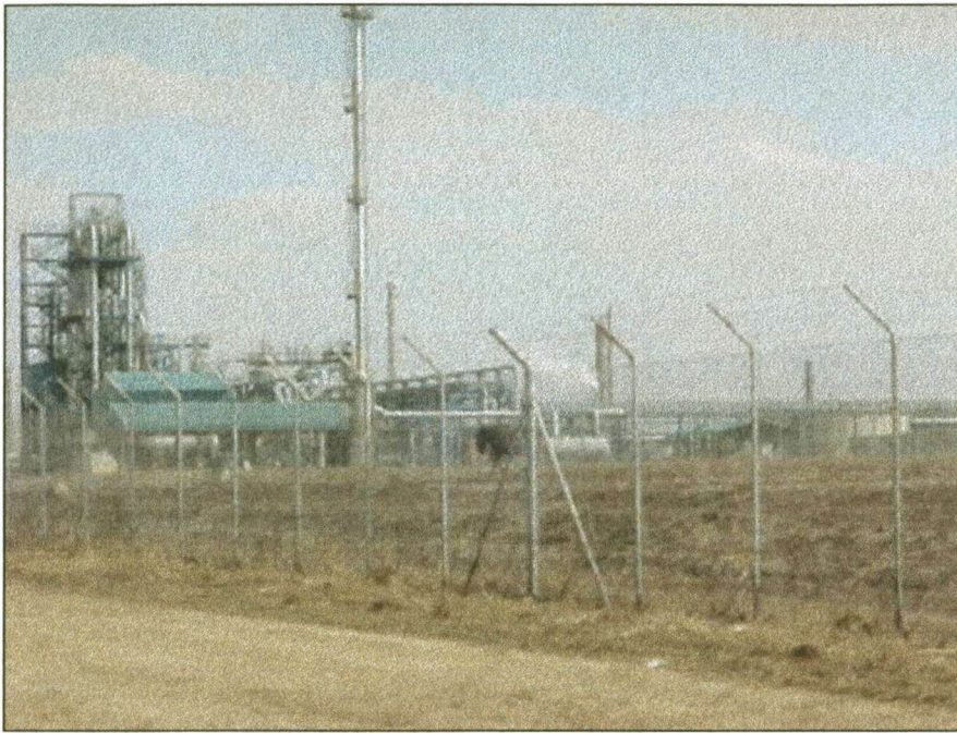
Figure 9: Poly 4 plant at the Safripol factory site.
