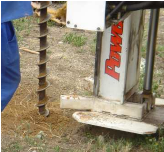
Figure 6-29: Solid-stem auger drilling on the site.
