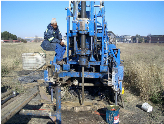
Figure 6-30: Drilling of Core hole GC1.
