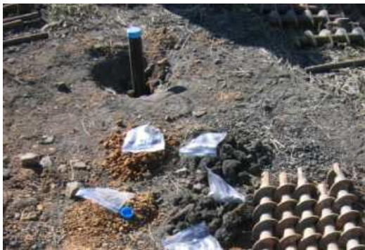
Figure 6-34: Piezometer drilled by solid-stem auger.
