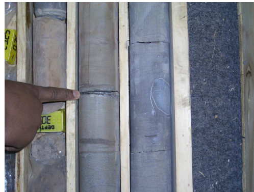
(f) Partially filled horizontal fracture
