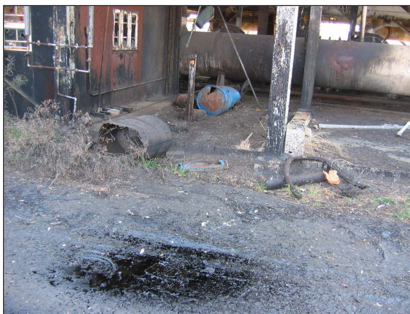
Figure 6-11: On-going spillage from tar loading.
