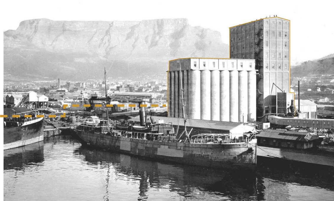
Fig. 72 The Grain Silo constructed in 1921 makes up an important part of Cape Town's skyline. (www.heatherwick.com, n.d.: Online)
