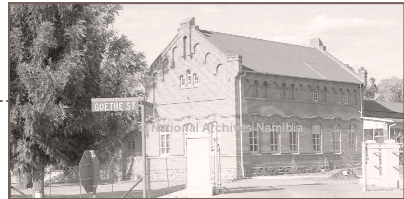
Fig. 36. (Above) Old High Court as viewed from Goethe Street, Windhoek. (1908-1909) Photograph: Schoedder, E. (1987)
