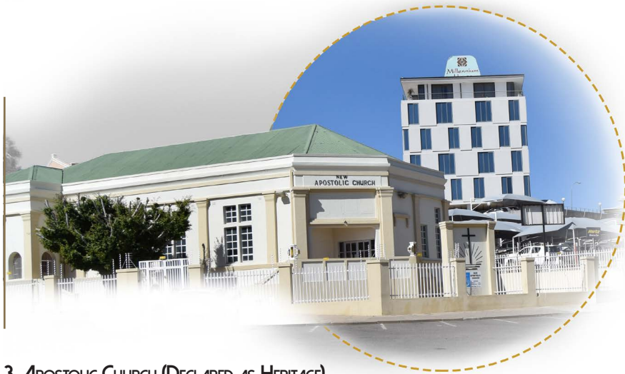
3. APOSTOLIC CHURCH (DECLARED AS HERITAGE) AND MILLENNIUM HOUSE CORPORATE BUILDING
