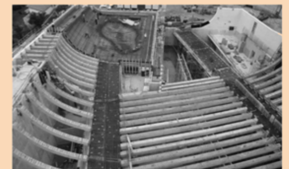
(Figure 81. Roof Structure, Museum of ocean and surf, 2020)
