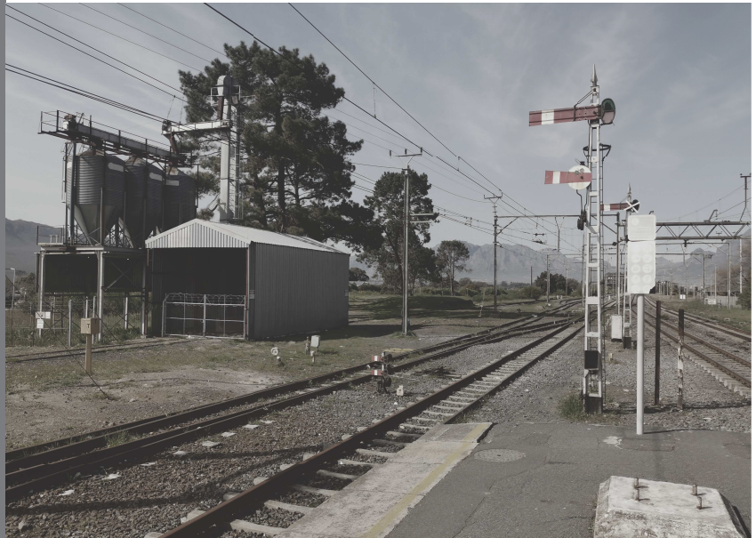
Figure 18: Photo of existing train maintenance workshop (Out-of-service), to be transformed as an attempt at architectural re-use. (Haasbroek, 2022).
