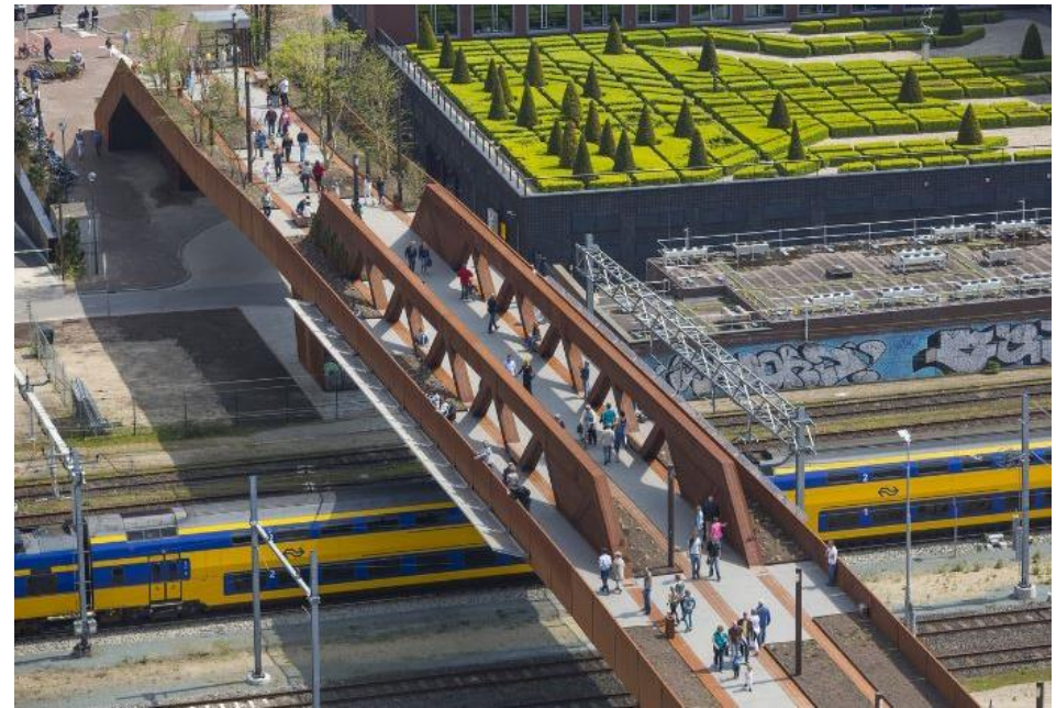
Fig 102: Truss-like structures on Bridge (Linders, undated)
