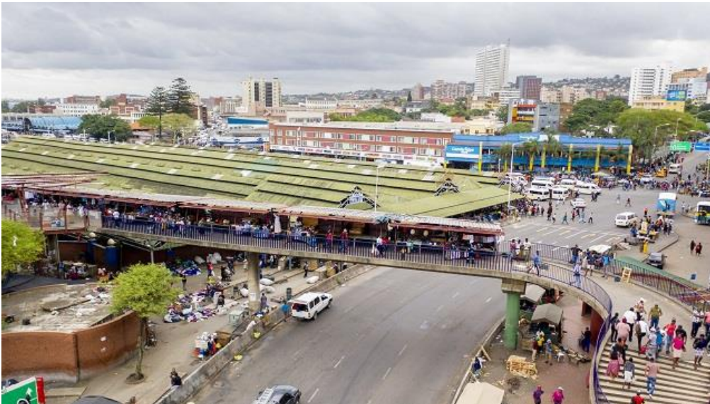
Fig 48: Warwick Junction, Durban (Galvin & Maassen, 2019)
