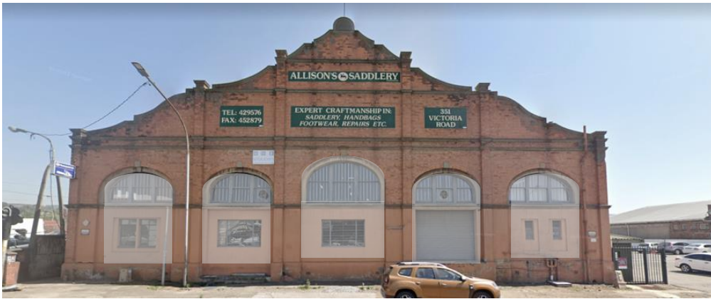
Fig 57: Windows to be replaced (Author, 2023)
