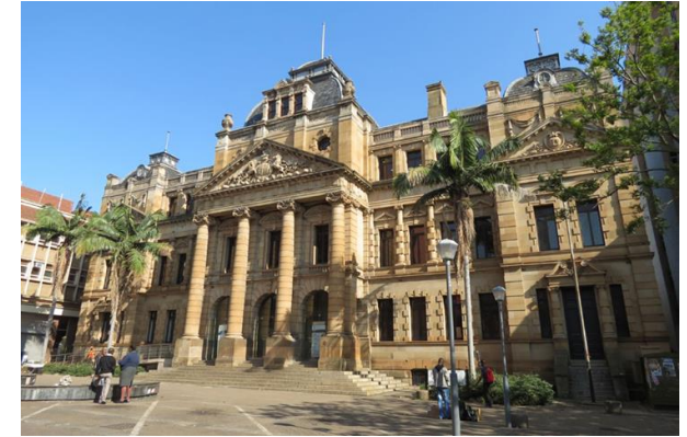
Figure 10 :Old Colonial Building (SA-Venues, undated: online)
