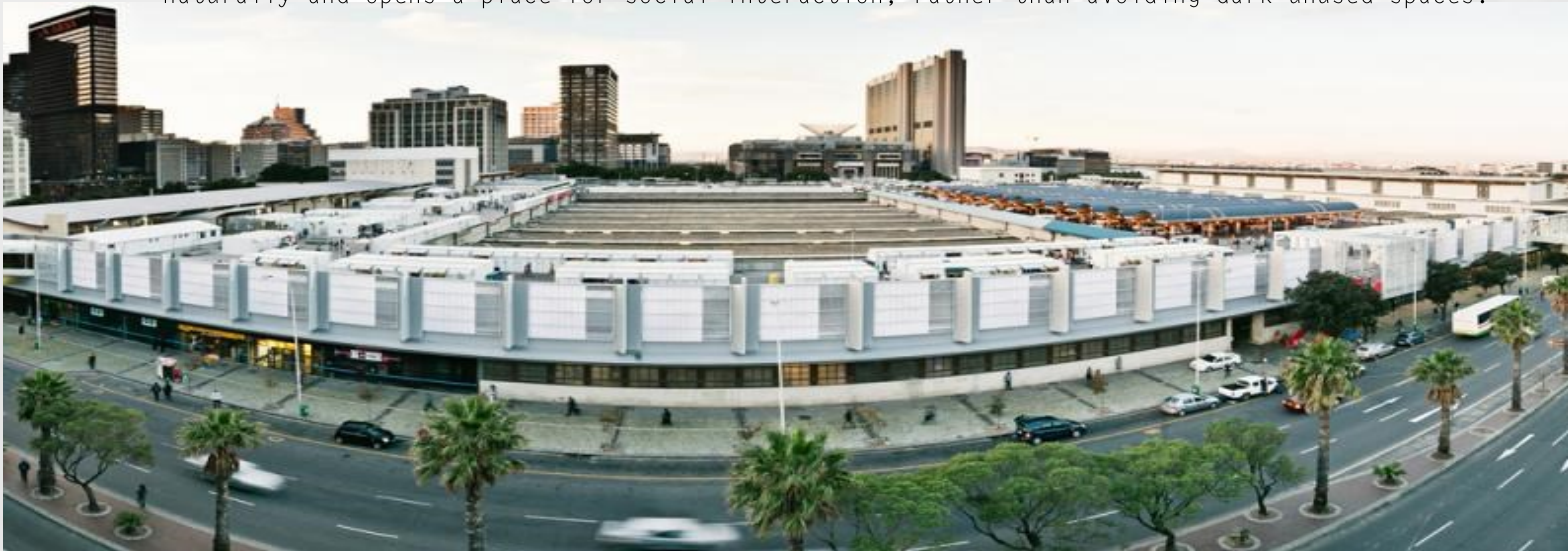
Figure 31: New Strand Road Façade for Cape Town Station. By Architects. 2012
