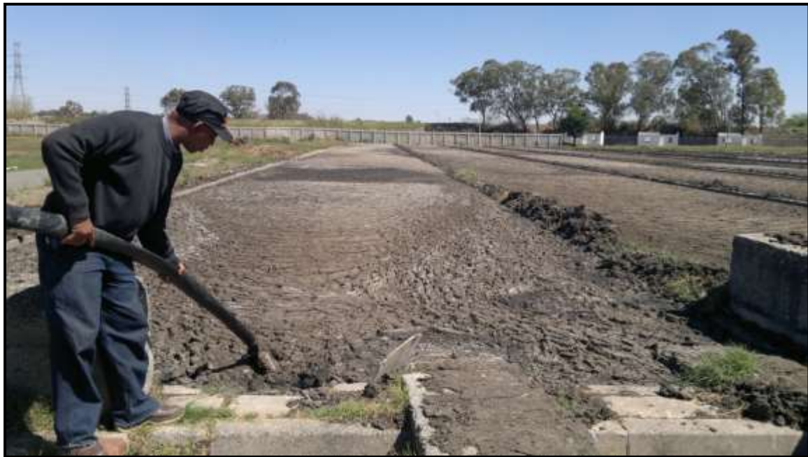
Figure 6.2 The sewage works in Bloemfontein (b).
