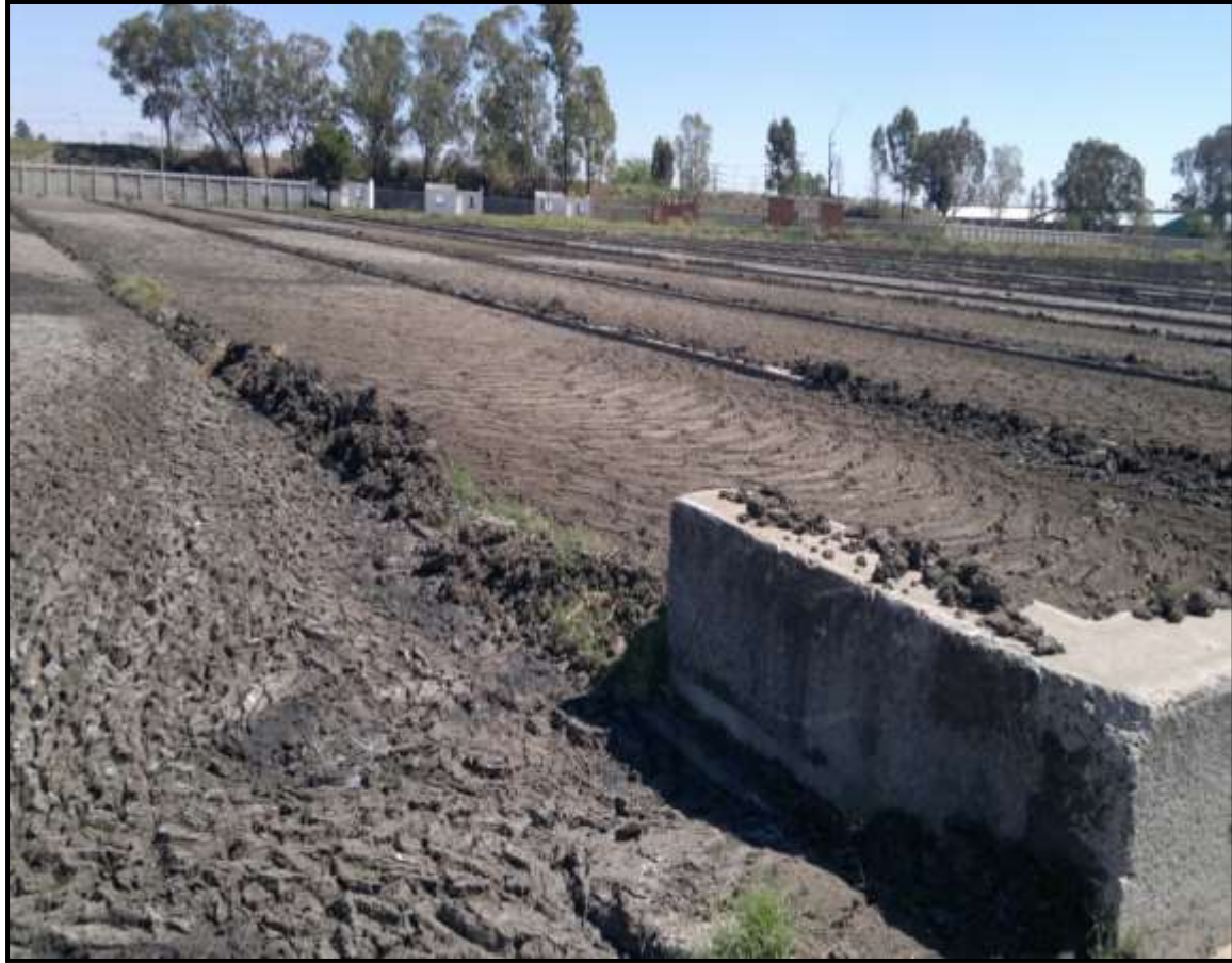
Figure 6.1 The sewage works in Bloemfontein (a).
