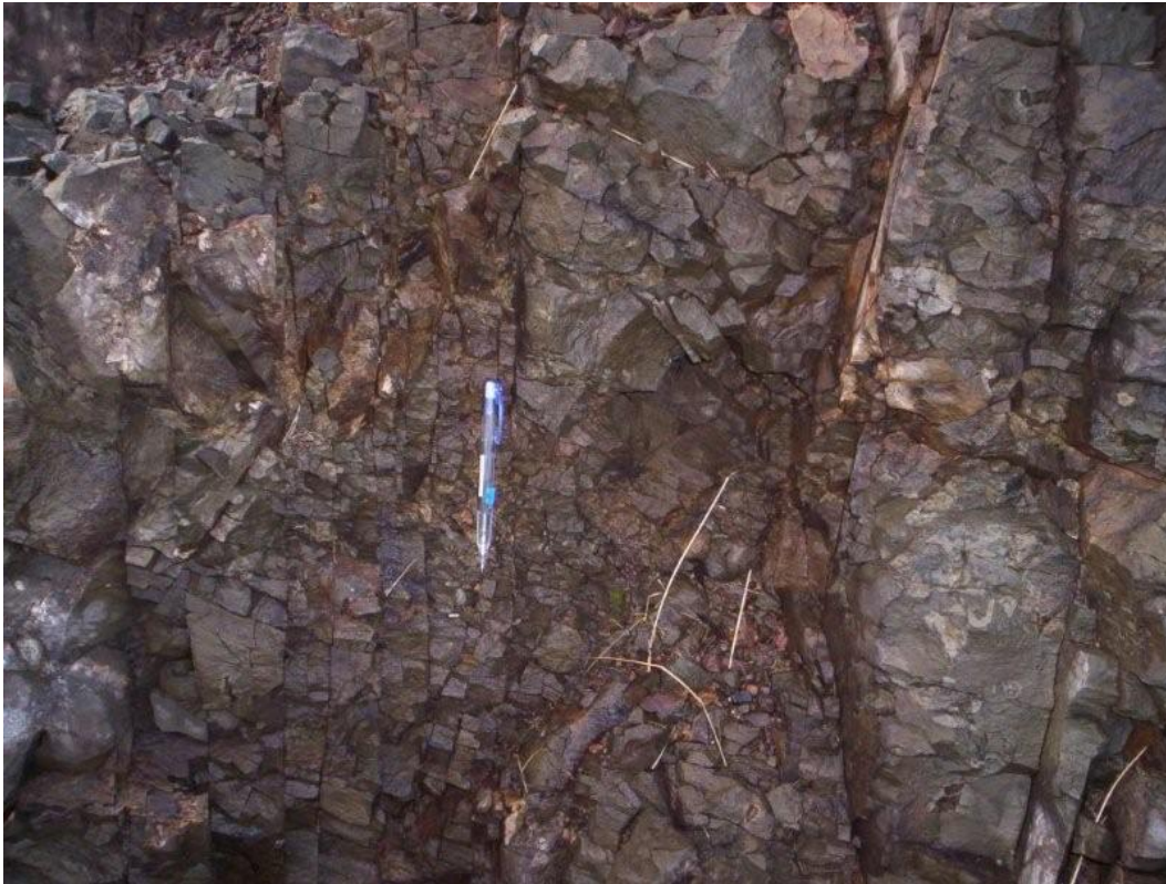
Figure 4-9 Weathered mudstone on the footwall of the Beaufort West sill
