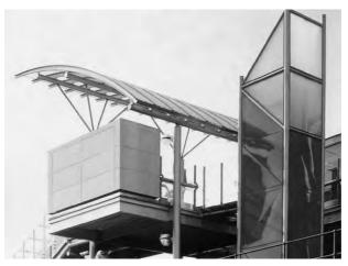
Figure 7: Dockland Light Rail Station. Designed to be used as a kit of parts for all stations.
