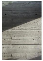
Figure 125: Board marked finish - the result
