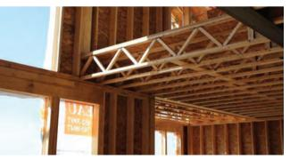
Figure 110: Wood Floor rafter System
