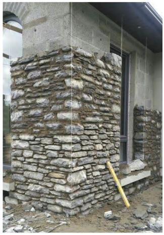
Figure 117: Addition of stone cladding on to cinder block walls
