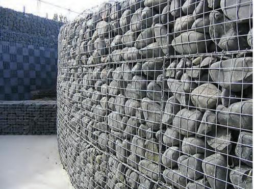
Figure 124: Completed Gabion Wall
