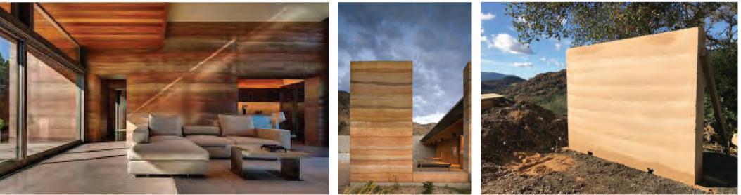
Figure 100: Interior Structural usage of rammed earth
