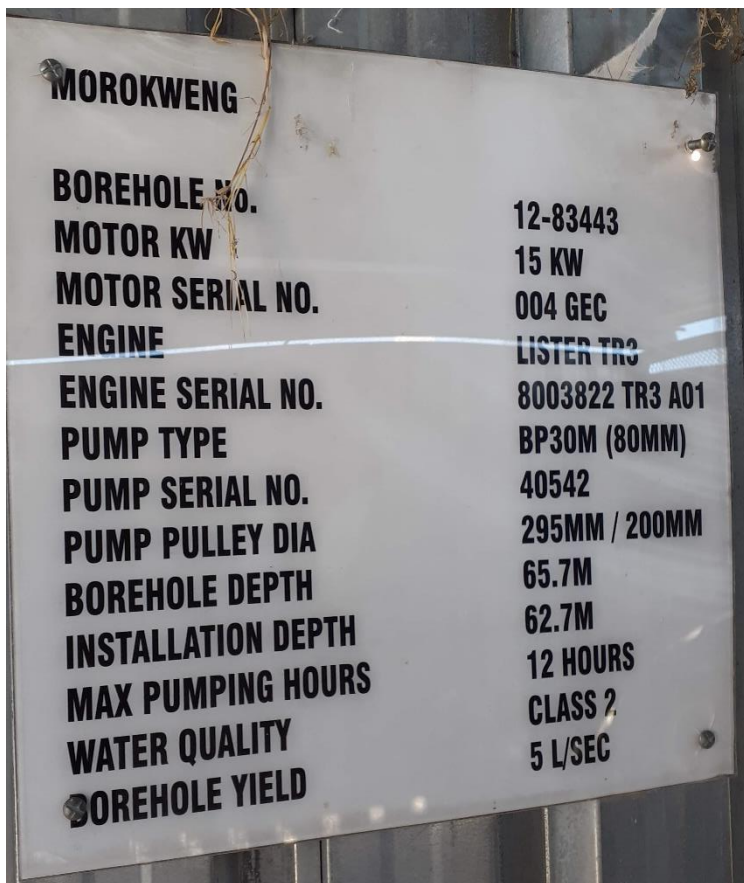
Figure 7.6 Borehole 12-83443 information board
