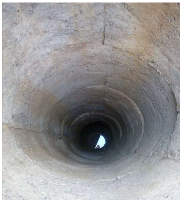
Figure 2.13 Unscreened concrete-lined large-diameter hand-dug well
