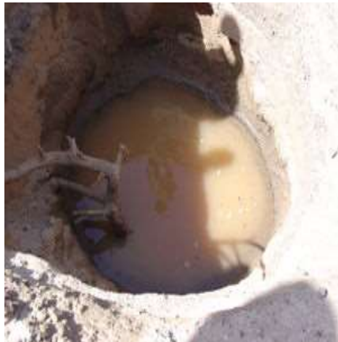
Figure 2.5 Unlined large-diameter well with contaminated water seeped in through the soil
