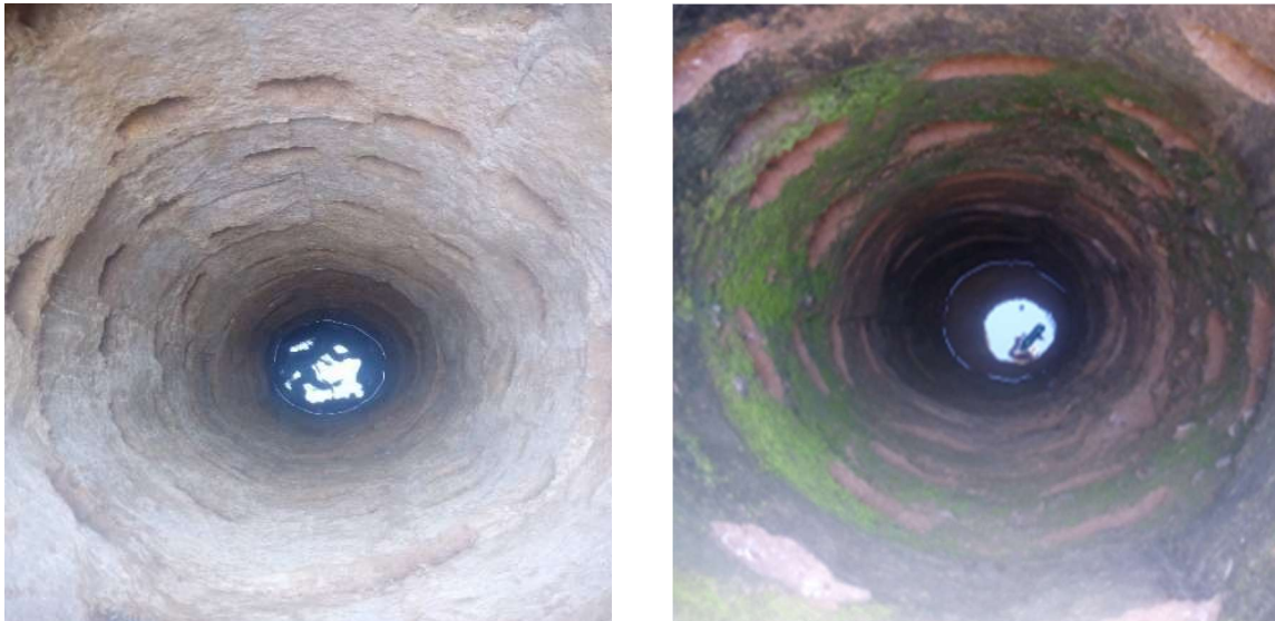
Figure 5.2 Screened-lined large-diameter hand-dug wells at test site
