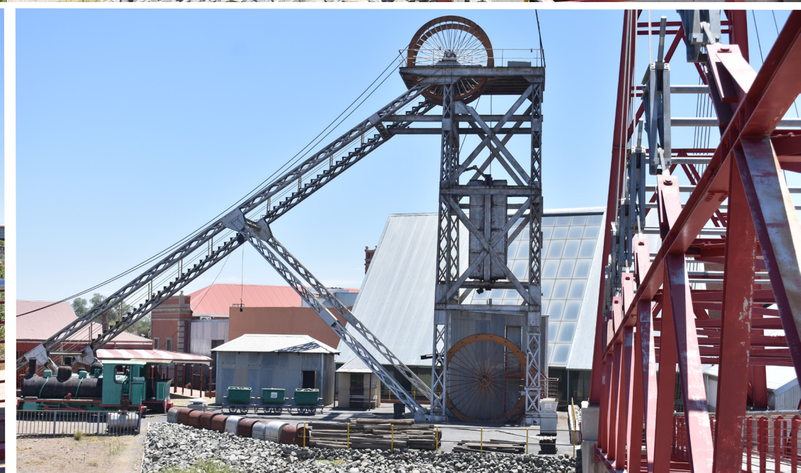
Figure 75: Kimberley Mine Headgear
