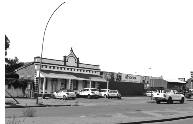
Figure 63: Youth Development Centre to the East of the Site
