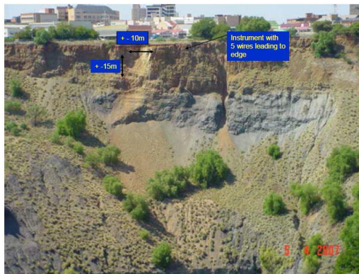
Figure 164: Photographs of mine damage (Maree, 2017)
