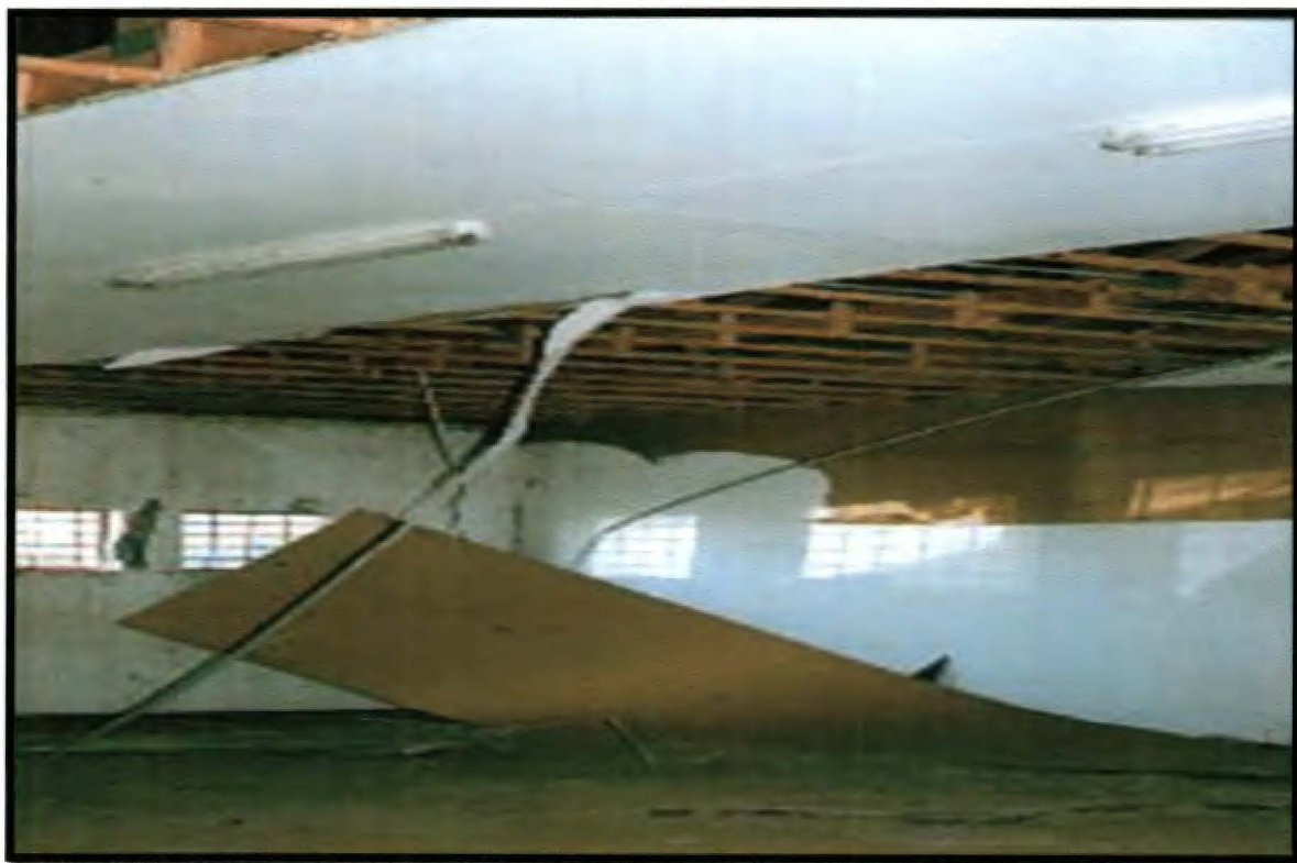
Photo 5: Vandalized Business Units in Tseki and Makeneng Shopping centres
