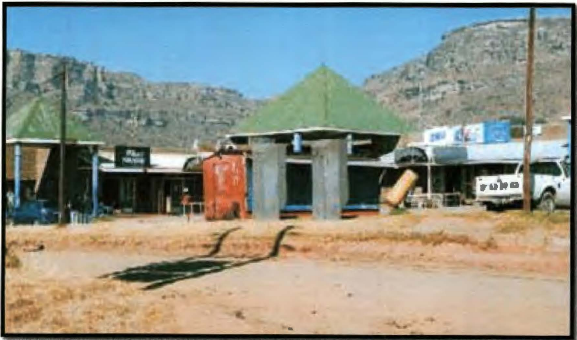
Photo 1: Monontsha Shopping Centre with no fence
